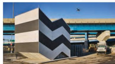
Located by the Van Wyck Expressway, within a Department of Transportation maintenance yard that is a refueling site for DOT vehicles, this diesel monitoring booth is chevron-shaped in plan and includes a bent ribbon window that captures a panoramic view of the yard. The booth's facades light-heartedly reference traffic symbols and road markings with alternating black and white glazed tile cladding set in a supergraphic zig-zag pattern with 'Safety Yellow' accents.
