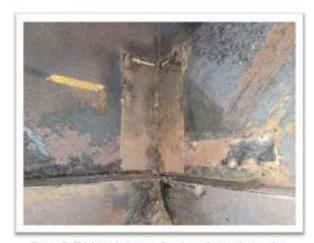
Figure 7. Thickened corners showing advanced corrosion
