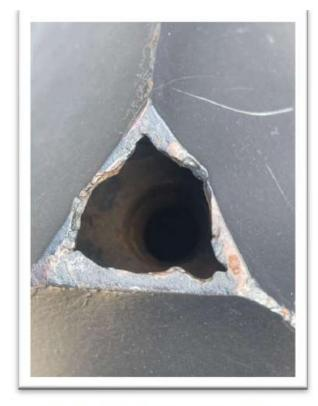
Figure 5. Top of Cube, missing cover
