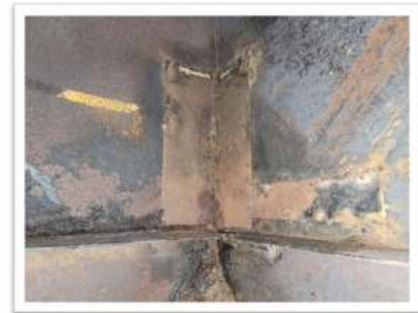
Figure 7. Thickened corners showing advanced corrosion
