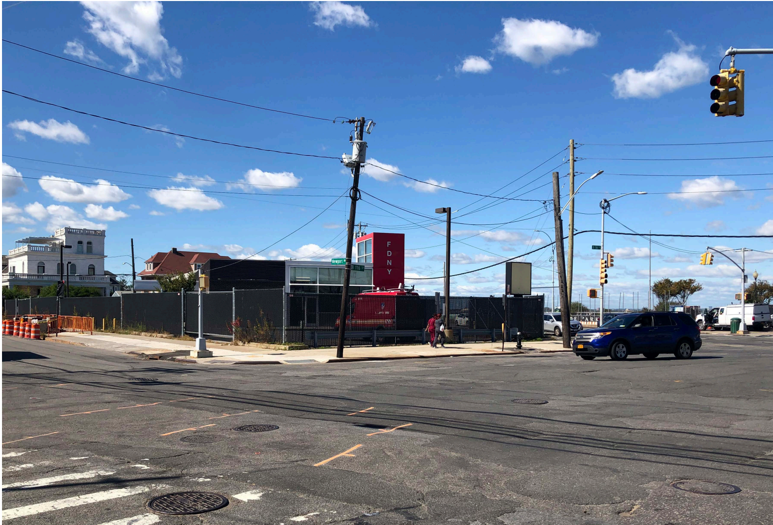
1 - View from Beach 116th St. (existing bank building)
