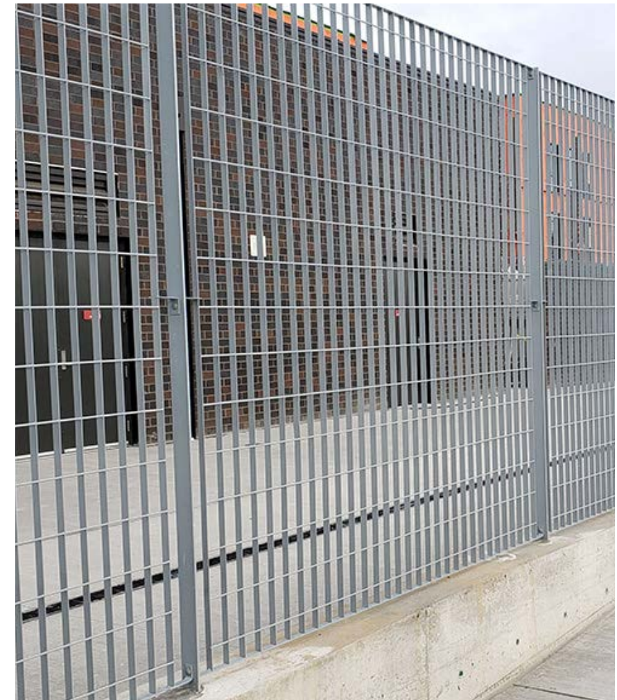
Rectangular grid panels, gray color powder-coated steel
