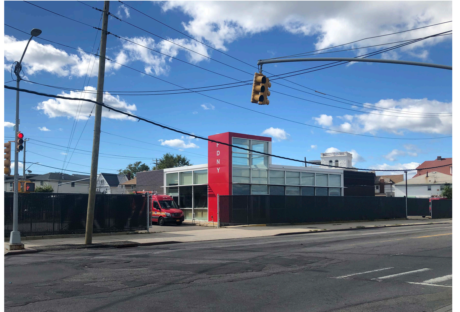
2 - View from Beach Channel Drive (existing bank building)
