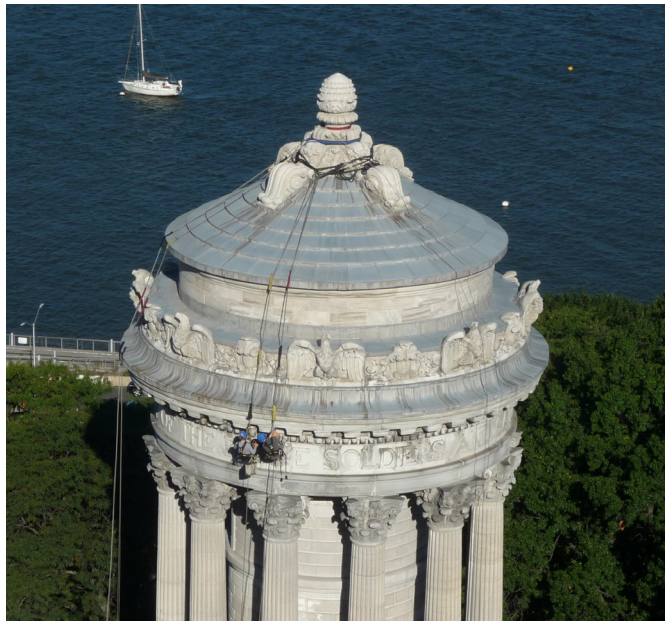
Main Roof and the Entablature
