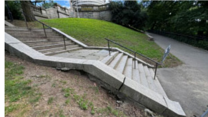
Northwest stairs and cheekwalls
