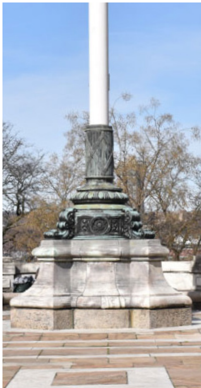
Flagpole Shaft Base
