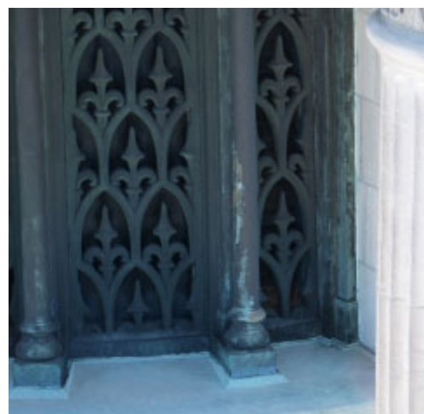
Window Grille on Drum
