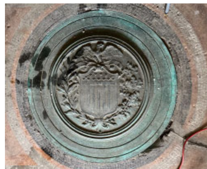
Interior Vault Manhole Cover
