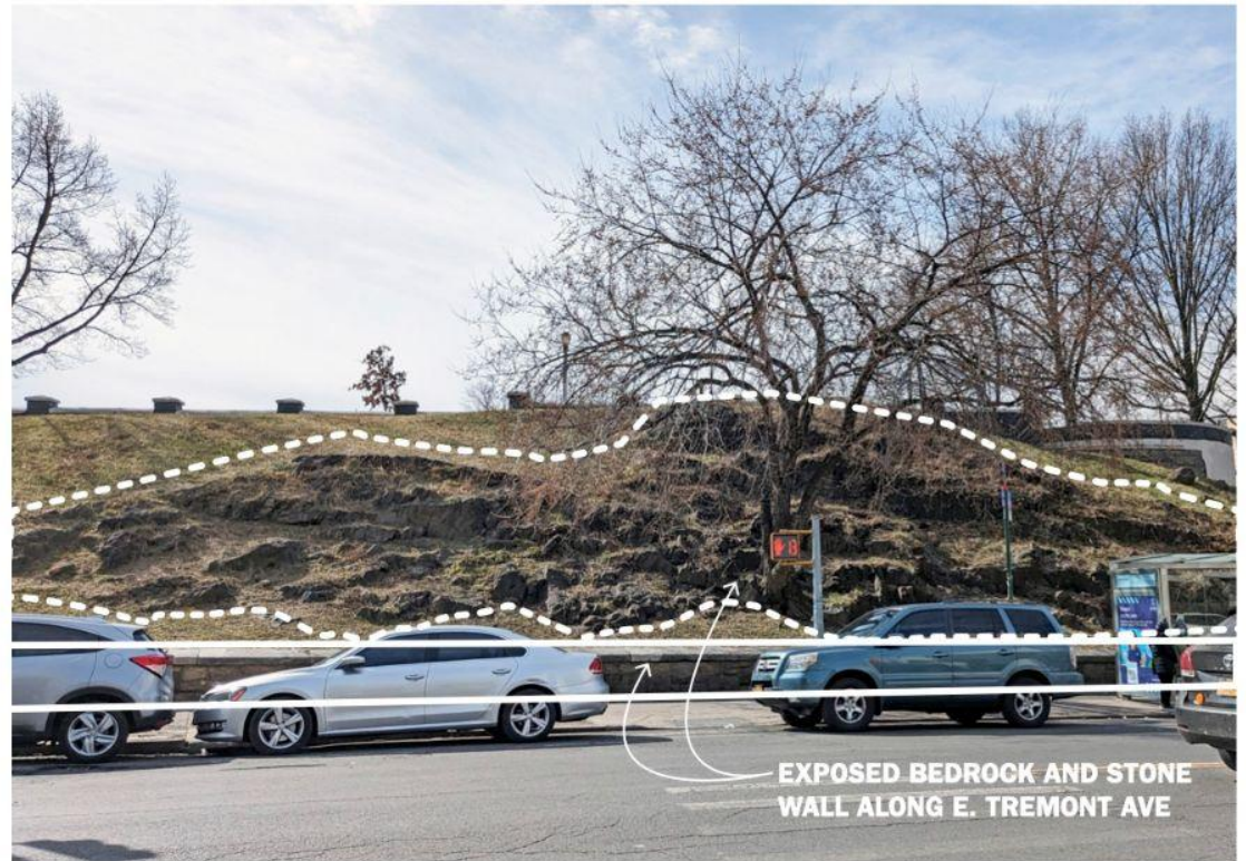
2 | View of exposed rock along E Tremont by project site
