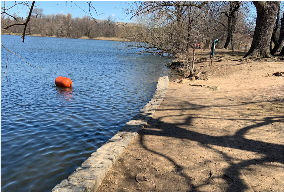
Broken retaining wall and eroded soil
