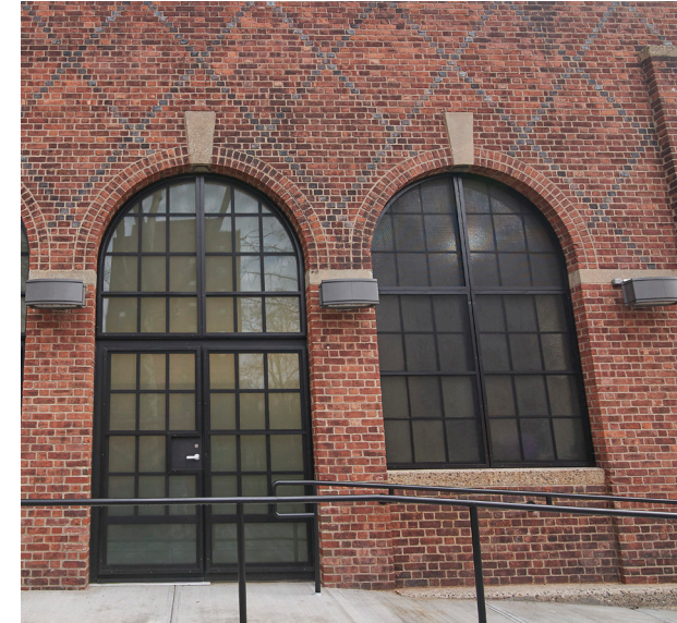
Steel door with security screens
