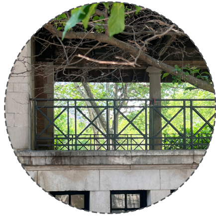
Original iron fencing
