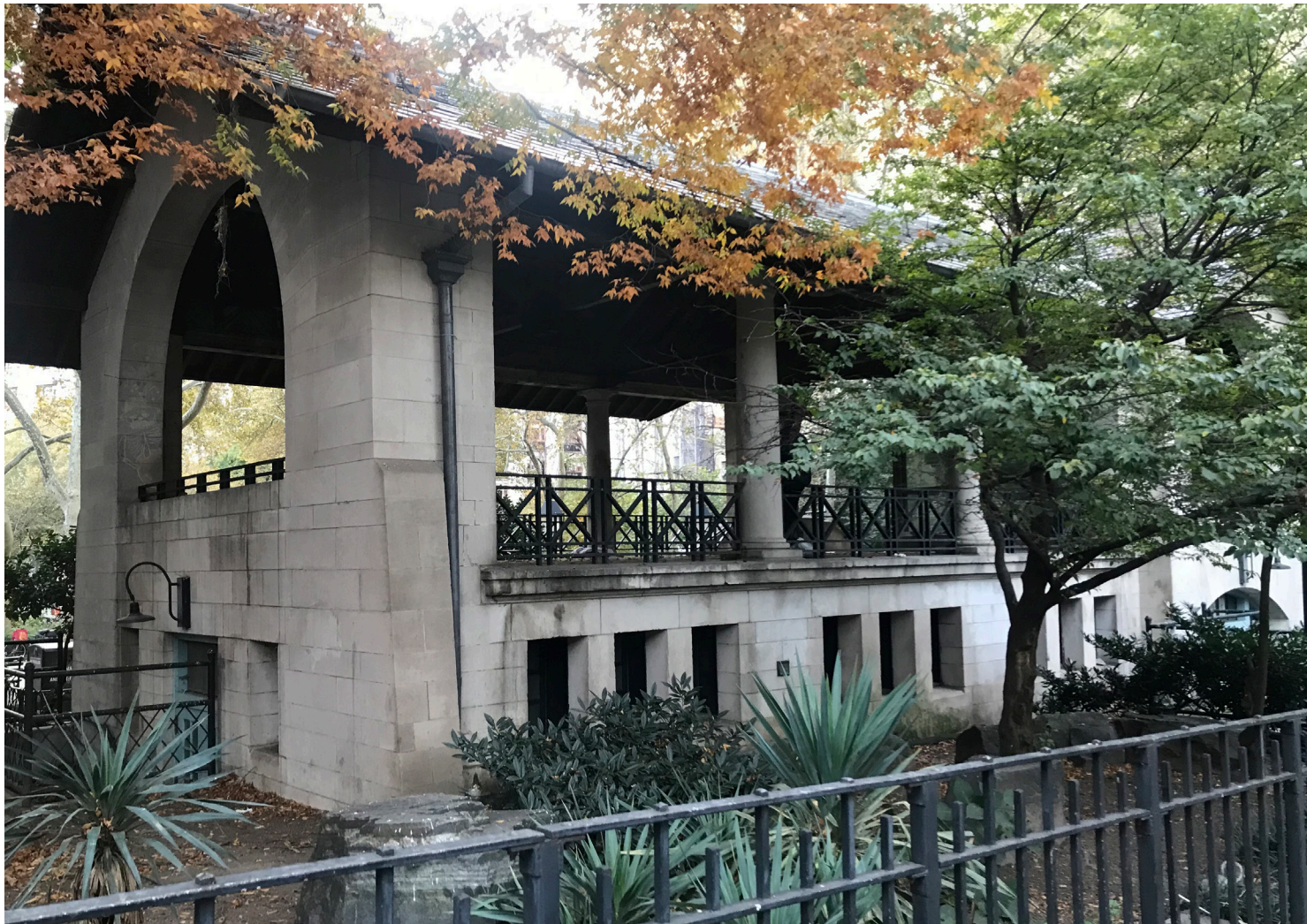
3- Pavilion ground floor view - Guardrails
