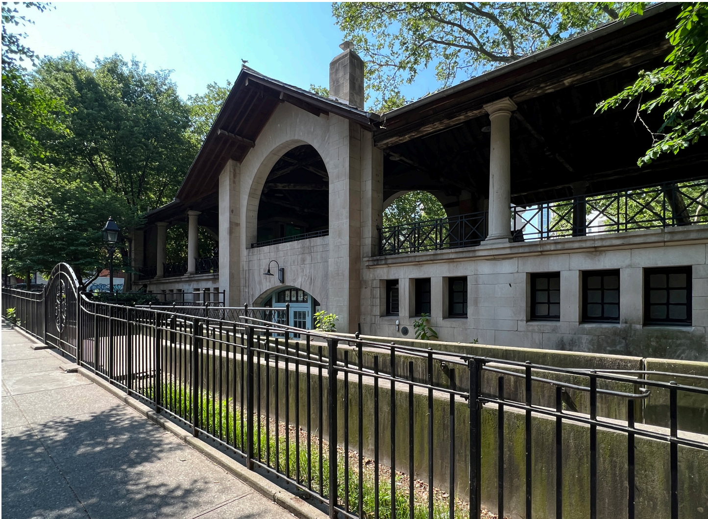
2 - Pavilion - North Facade
