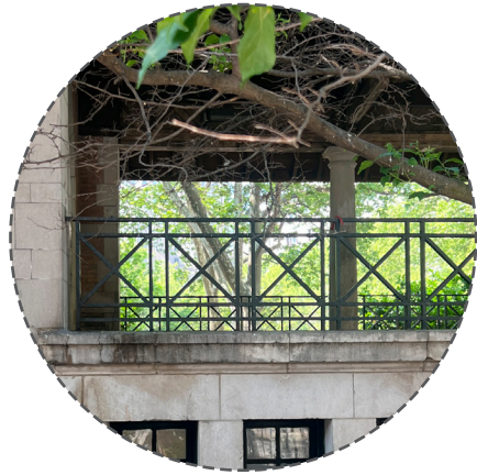
Original iron fencing
