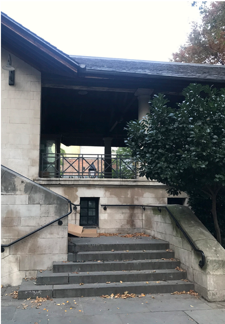
4- Pavilion ground floor view - South Stairs
