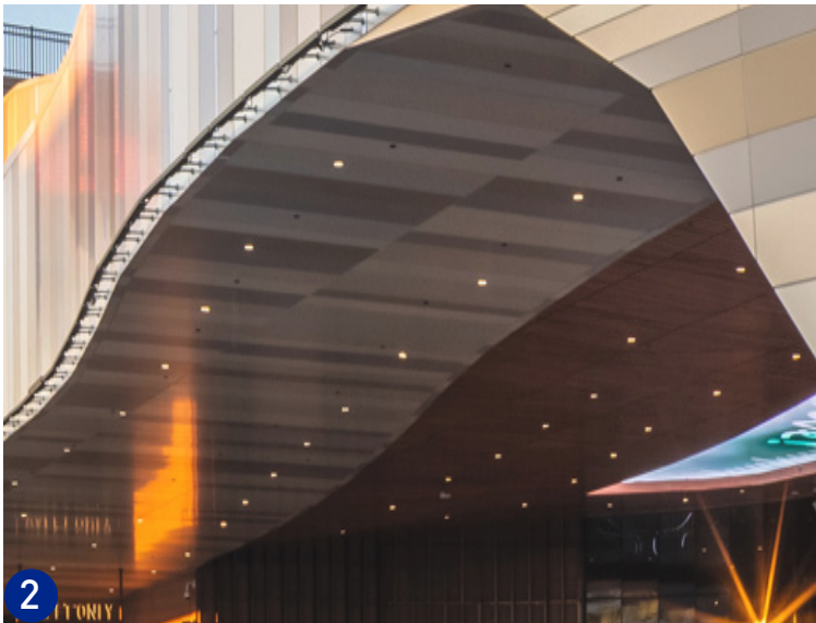
MATERIAL METAL PLANKING MANUFACTURER ALUCOBOND PRODUCT ALUCOBOND PLUS COLOR CADET GREY LOCATION @ SOFFIT + CEILING
