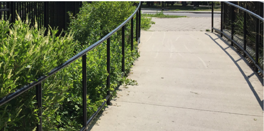
TYPE Poured Concrete LOCATION Walkways, Steps, Ramps, Curbs PROPERTIES Brushed Finish
