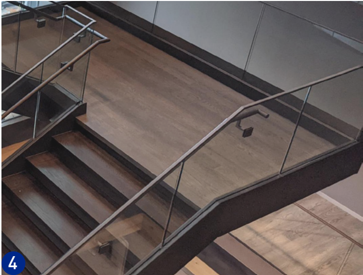
MATERIAL GLASS RAIL MANUFACTURER SIGHTLINE PRODUCT TRACK RAIL COLOR CLEAR LOCATION @ SOUTH PORTAL
