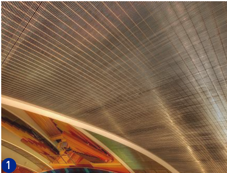
MATERIAL WIRE MESH MANUFACTURER BANKER WIRE PRODUCT RIDGE-FLAT THREAD FLEXIBLE MESH COLOR ALUMINUM IN ANODIZED GOLD LOCATION @ CLADDING
