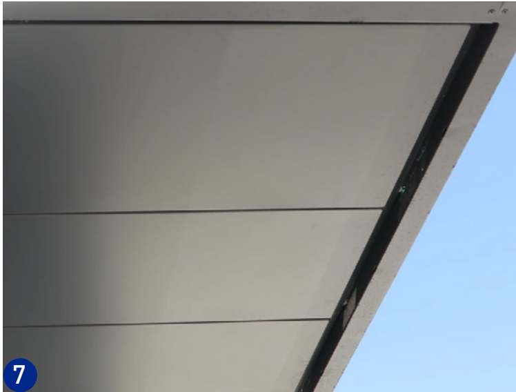
MATERIAL METAL PANEL MANUFACTURER ALUCOBOND PRODUCT ALUCOBOND PLUS COLOR GREYHOUND LOCATION @ SLAB EDGE
