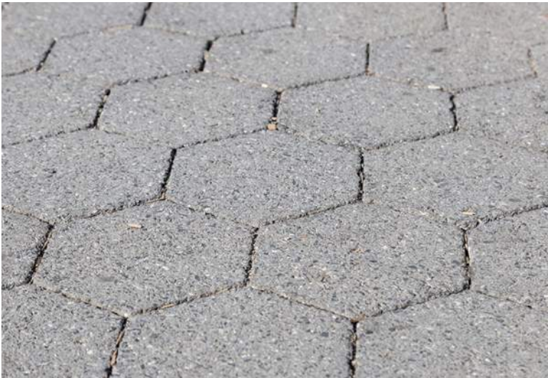
Asphalt Block Unit Pavers 8” Hexagonal Unit Pavers “Hanover Asphalt Block” by Hanover Architectural Products, or equal Finish: Ground Tudor Finish Color: A-80010
