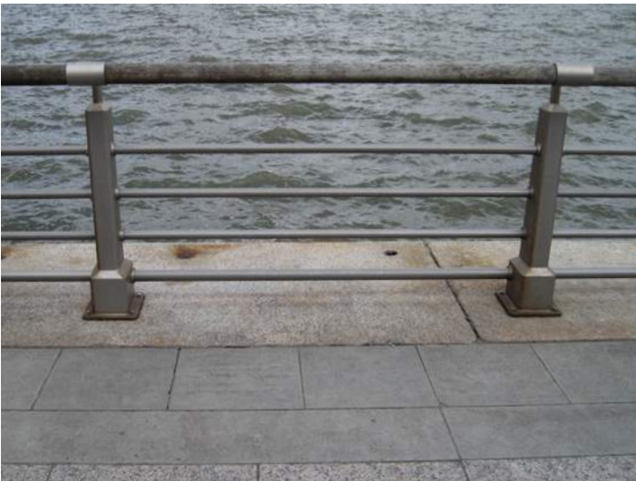
Stainless Steel Rails, Posts and Fasteners, Grade 316L
