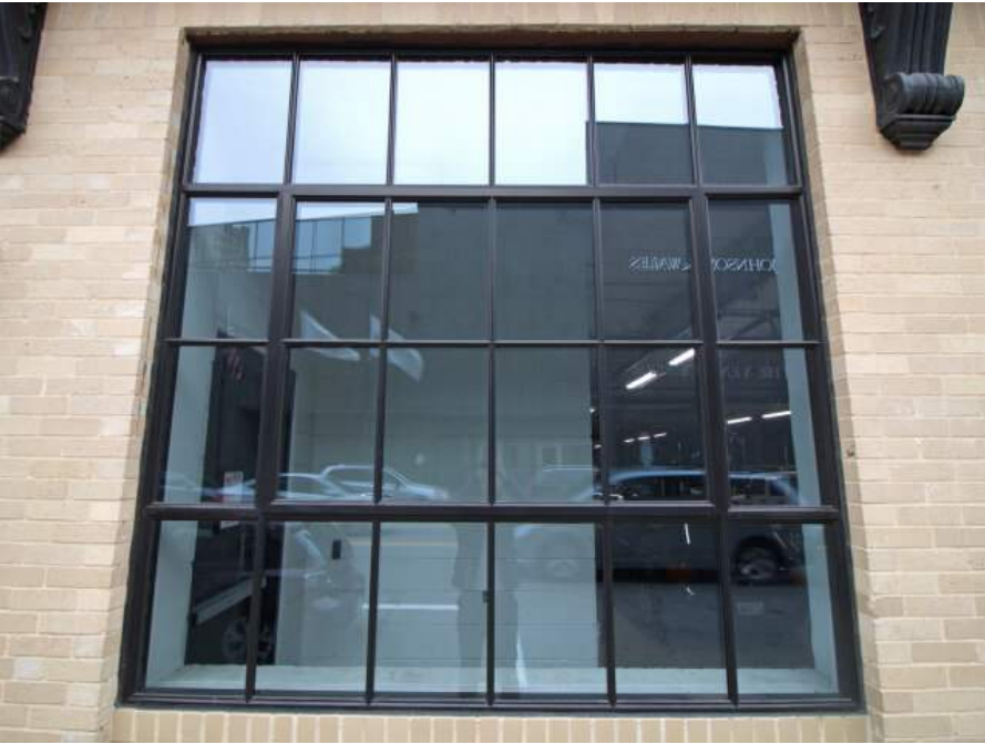
PIER SHED Level 01: Thermally broken Aluminum "Steel Replica" Windows
