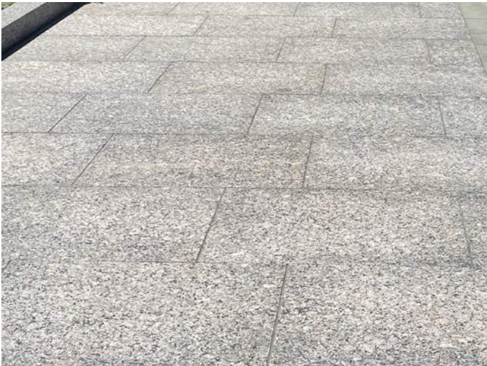
Granite Stone Material Type G-1 2” Thickness Finish: Thermal Color: “Autumn Brown” or “Polychrome” as quarried by Granicor, “Newton Brown” or “Huron Rose” as quarried by Polycor
