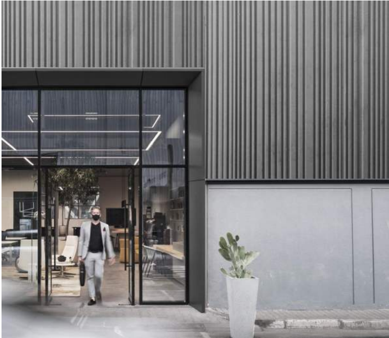
HEAD HOUSE Level 1 : Precast Concrete Panel Walls Ground Level : Cast-in-place Concrete Infill Walls
