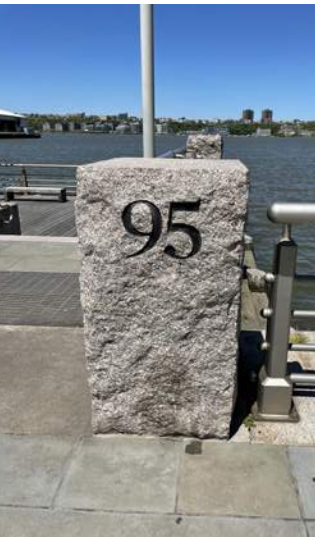
Granite Pier Marker, 2' Square Granite Post, 4' Height
