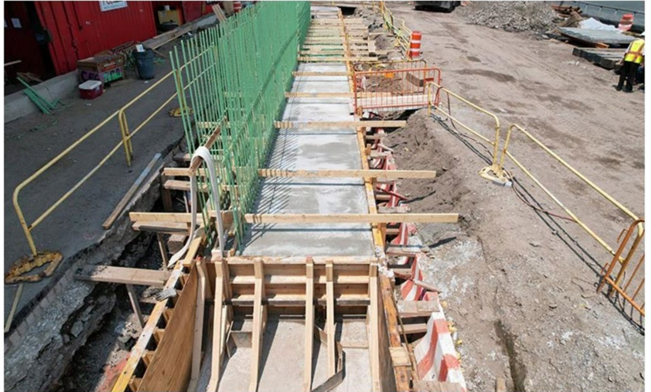
Wall foundation and formwork at Stuyvesant Cove Park, July 2021
