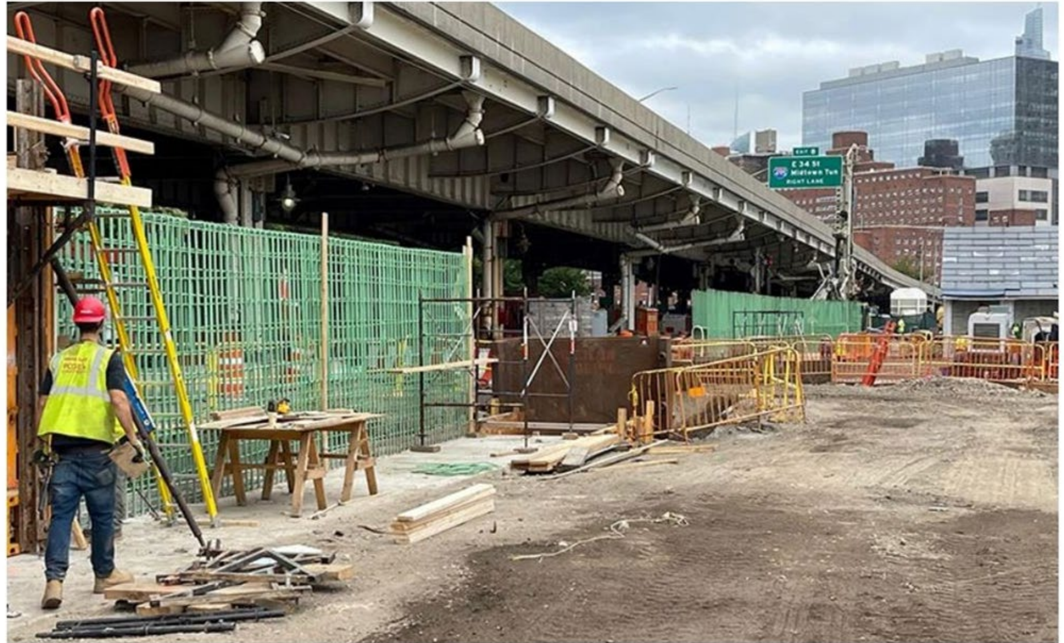
Rebar and formwork for floodwall at Stuyvesant Cove Park, July 2021
