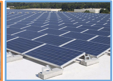
FLAT ROOF MOUNTED PV SOLAR PANELS WITH BALLASTS
