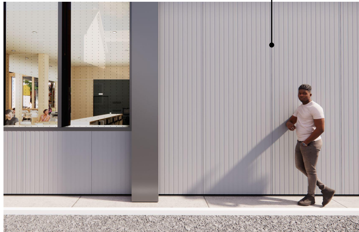
MTL-2 INSULATED METAL INFILL - KINGSPAN K-ROC
