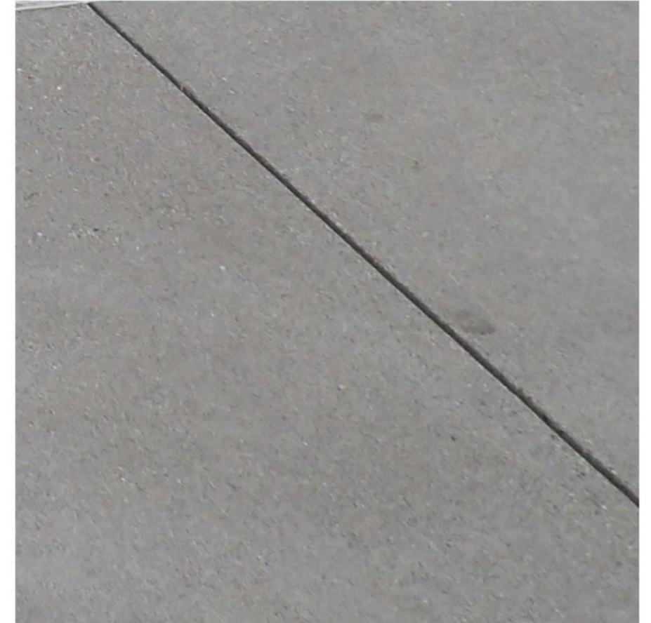
TINTED CAST IN PLACE CONCRETE - BROOM FINISH
