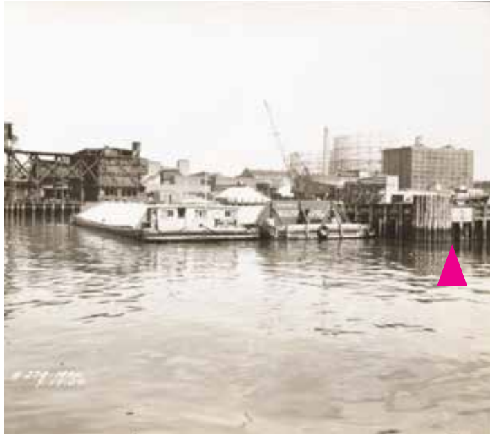
1934 East 107th Street Pier
