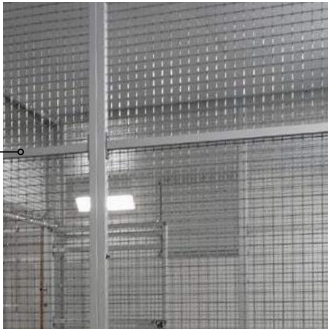
Porcupine Shelter Exterior Wall Caging: Galvanized mesh and tube frame
