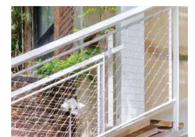
Guardrail Panel Web Net with Galvanized Rail
