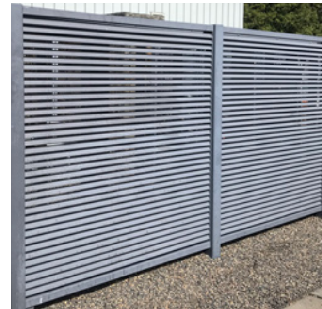
Black Powder Coated slatted metal screens to refuse store
