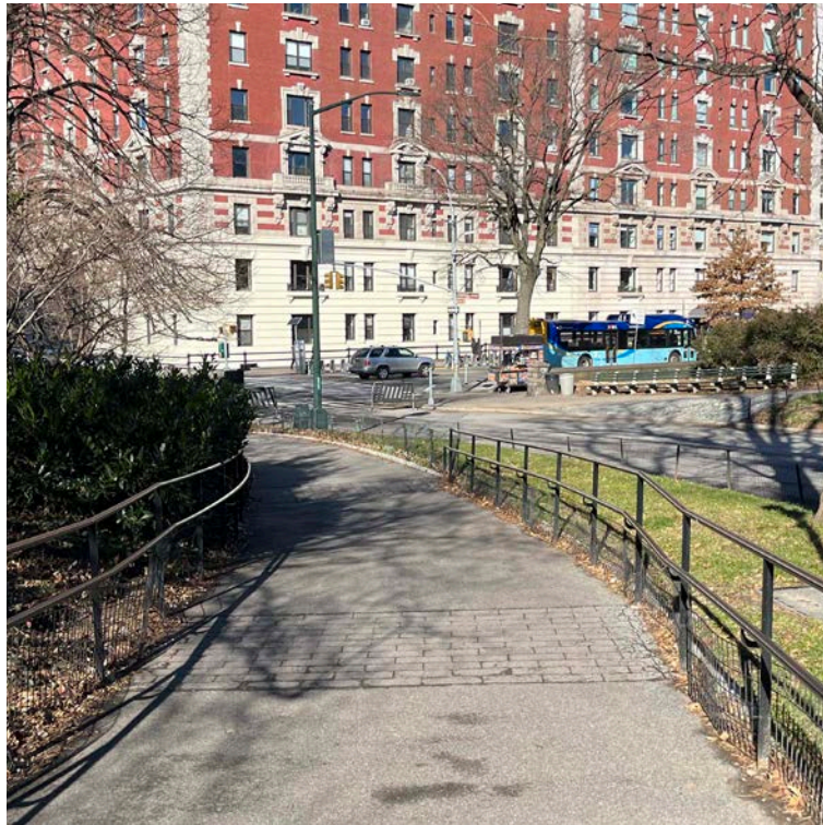
Accessible Path - Rectangular Asphalt Block Paver Landings and Child Handrail (Round Steel, Painted Black Finish)
