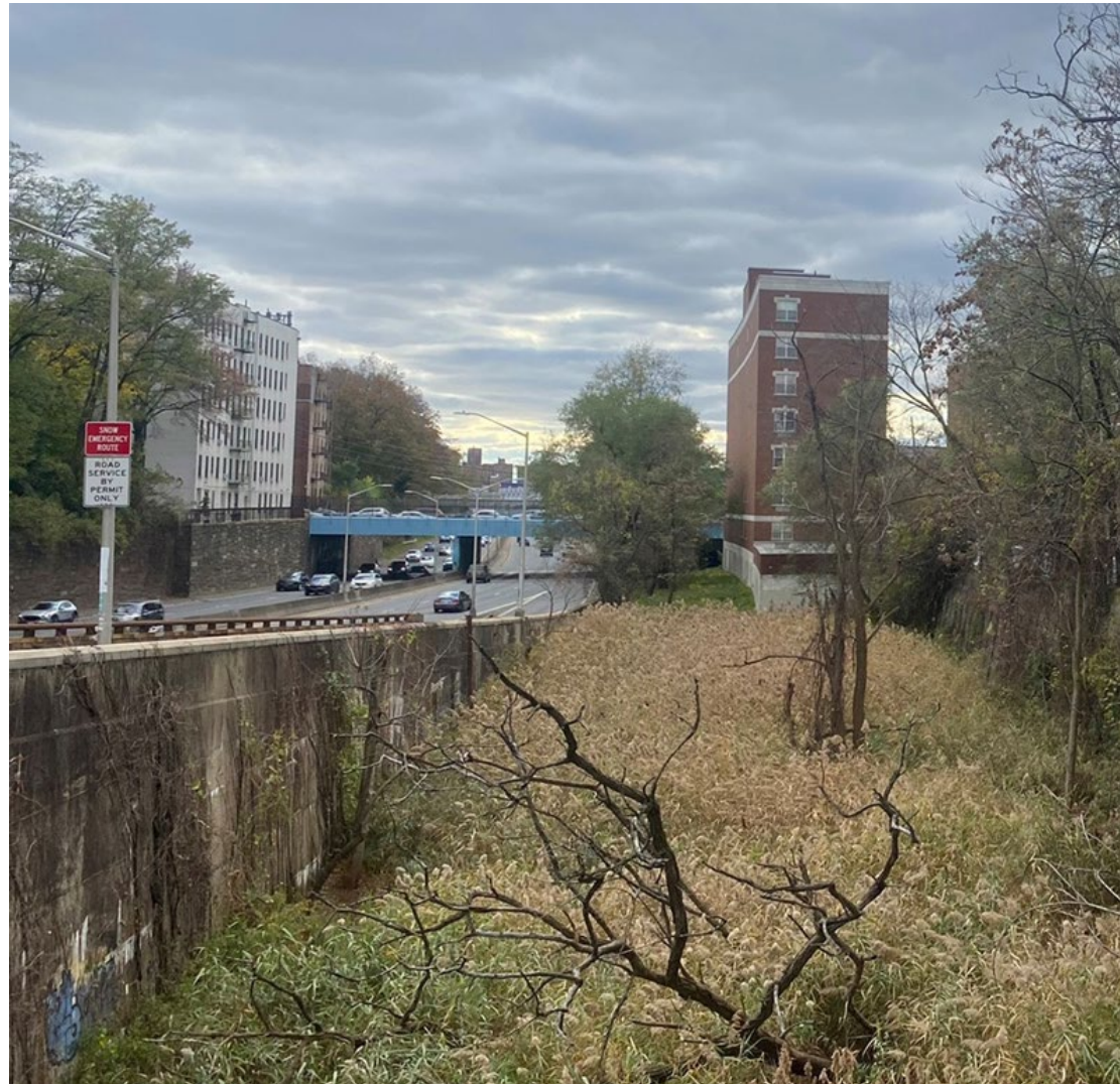
Current Conditions: W. 239th Street View Looking South
