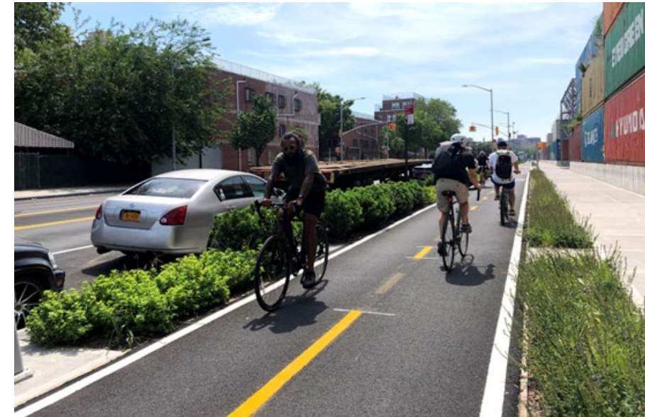
Kent Avenue, DOT/DDC Capital Project, 2021
