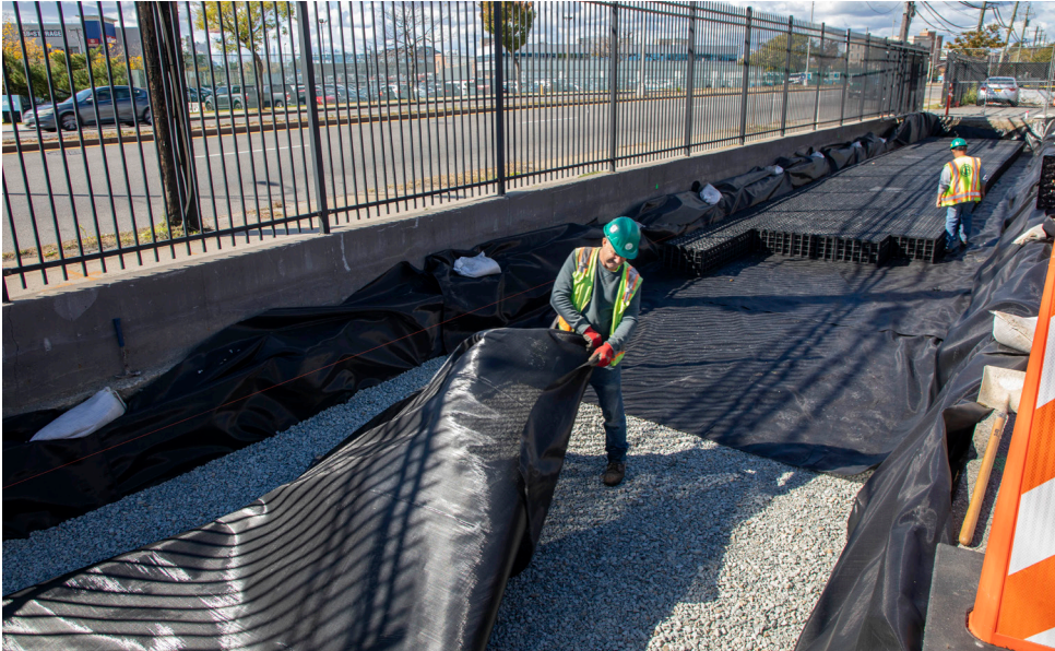
Subsurface storage system with gravel and retention crates during installation
