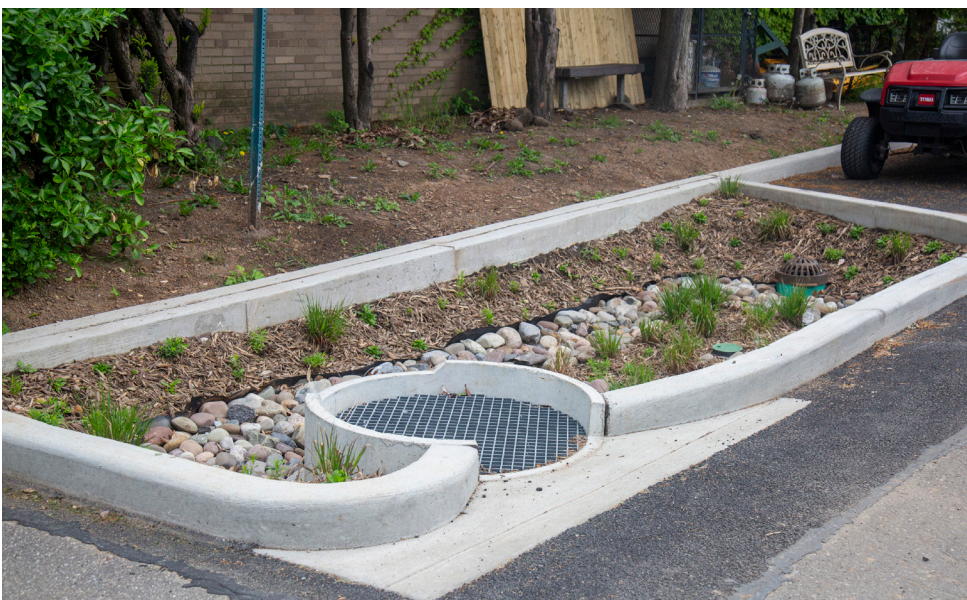
Bioretention feature draws stormwater runoff into subsurface storage system
