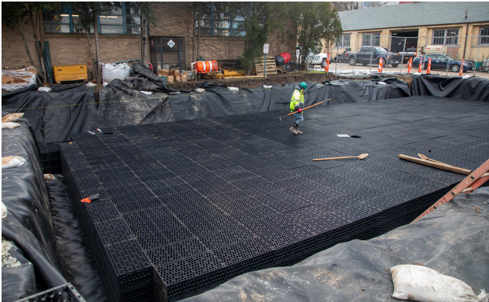
Subsurface storage system with retention crates during installation
