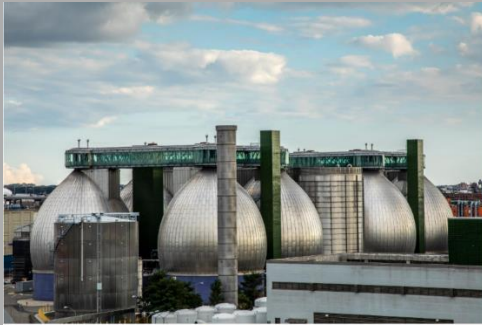
The New York City WWTB has eight unique Digester Tanks, which are like giant stomachs, digesting the sludge for several weeks.
