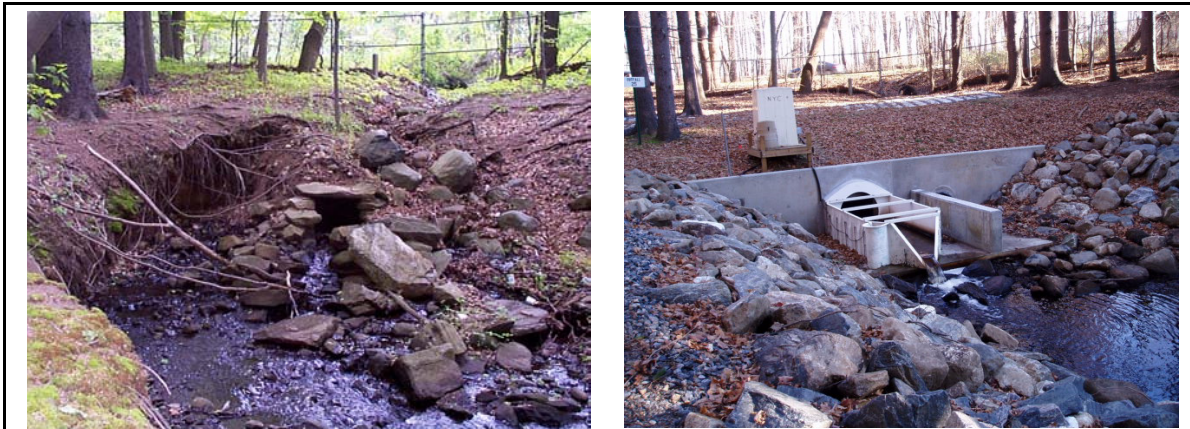
Figure 2.42 Photographs of Erosion Abatement Facility 68A.
