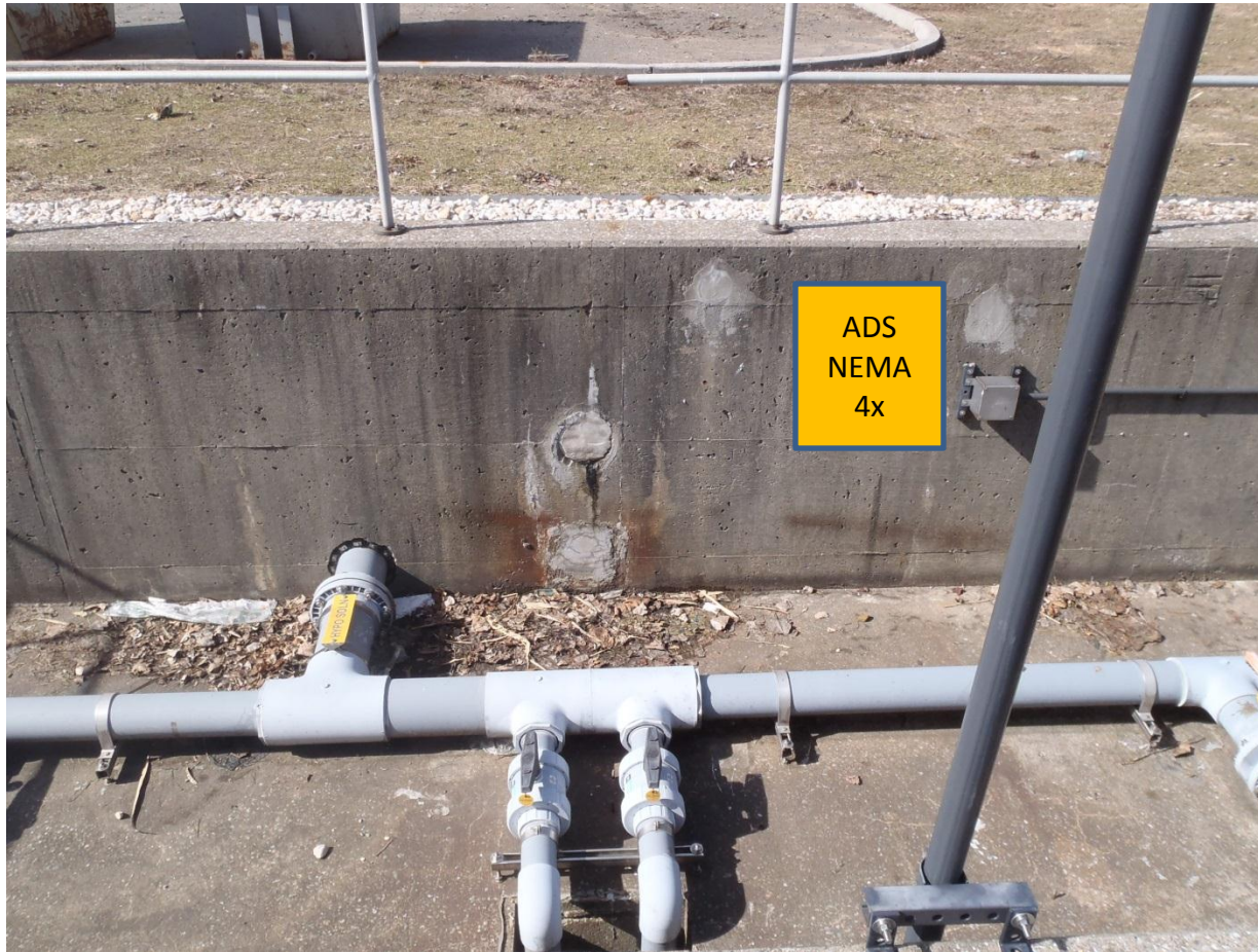
Photo 4 – East Meter Chamber and access point for temporary meters
