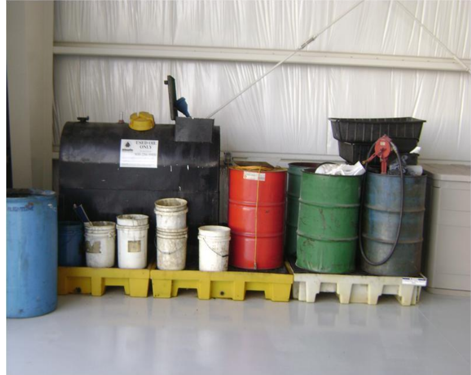
Lower Risk for Stormwater Impact: Drums stored indoors on spill pallets
