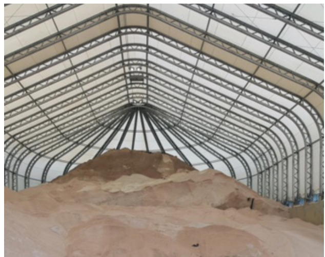
DSNY salt shed
