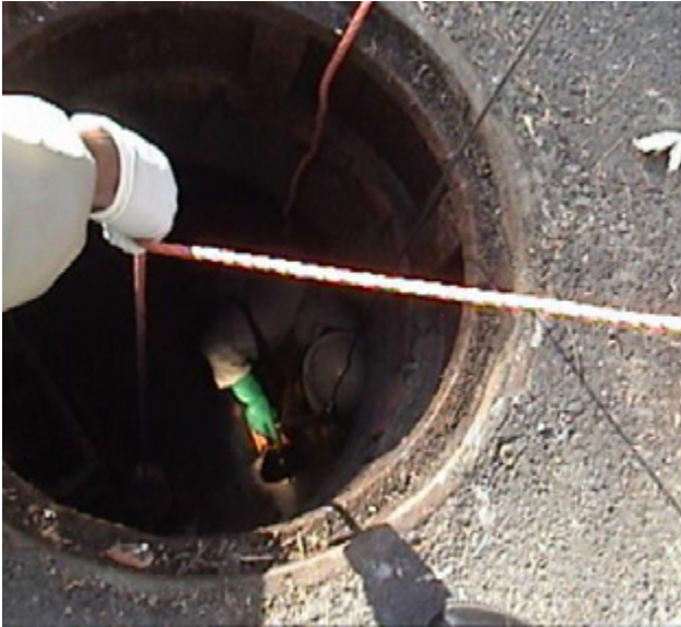
DEP staff begins sewer investigation
