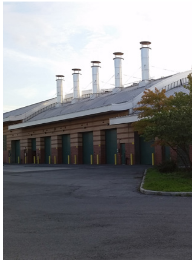
Paerdegat Basin CSO facility
