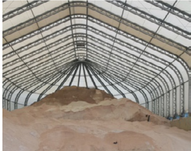
DSNY salt shed
