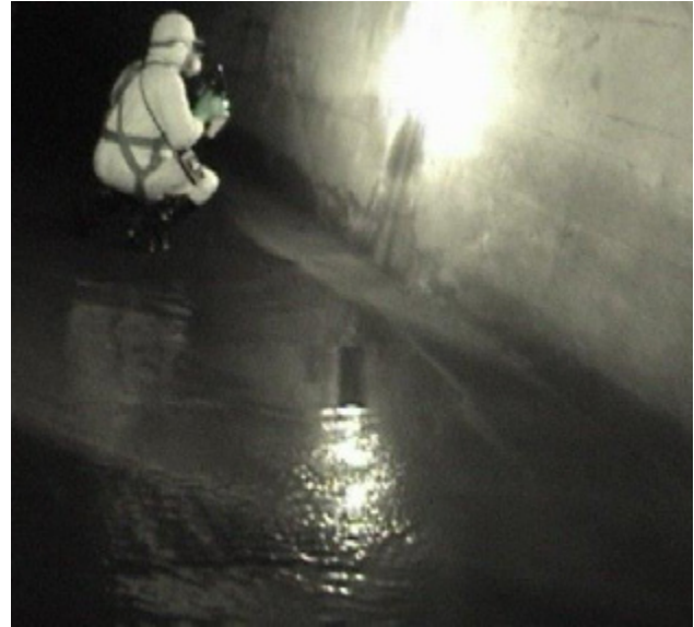
DEP staff conducts in-sewer investigation
