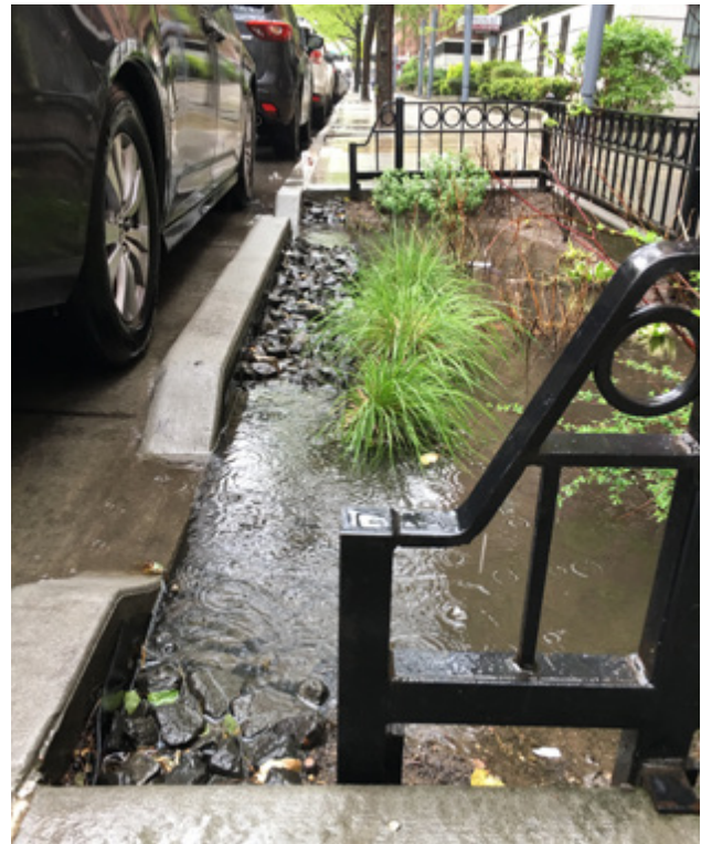
Rain garden construction in Flushing, Queens
