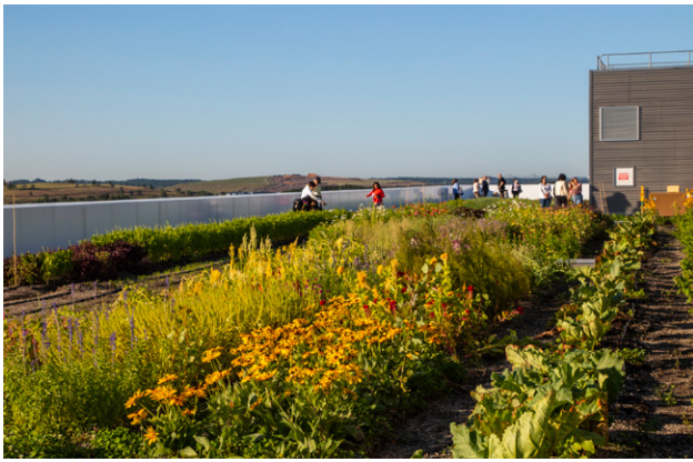
Rooftop retrofit at Corporate Commons Three in Staten Island.
