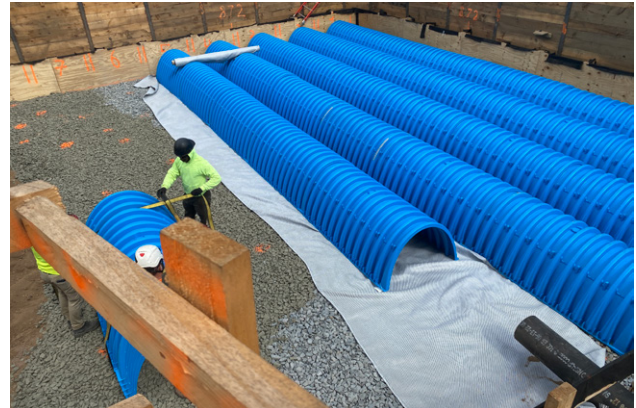
A subsurface retention practice at K095: Gravesend during construction.
