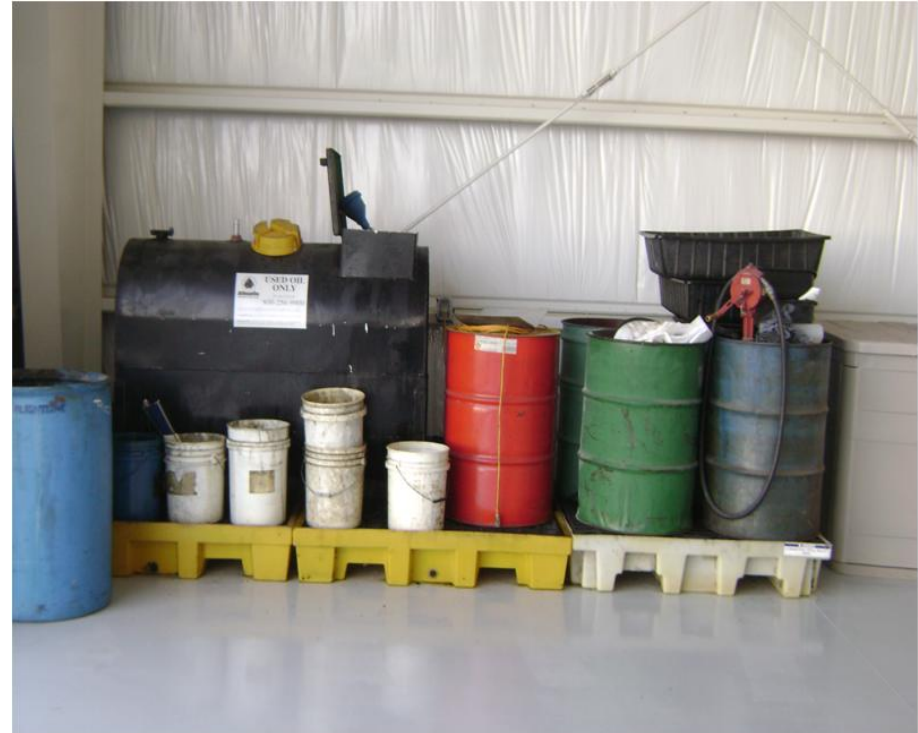
Exhibit B: Lower Risk for Stormwater Impact: Drums stored indoors on spill pallets
