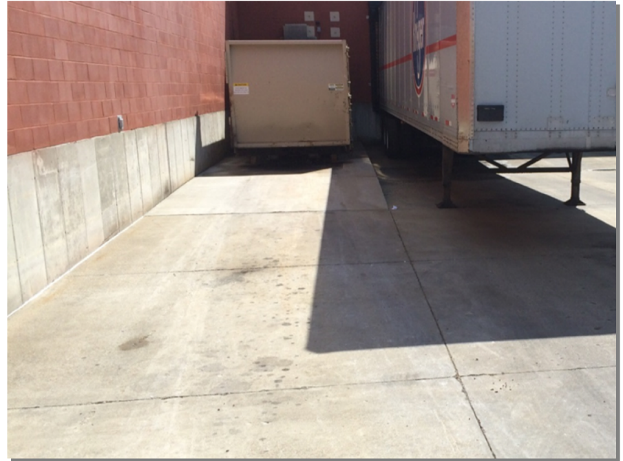
Exhibit B: Lower Risk for Stormwater Impact: Well-managed dumpster
