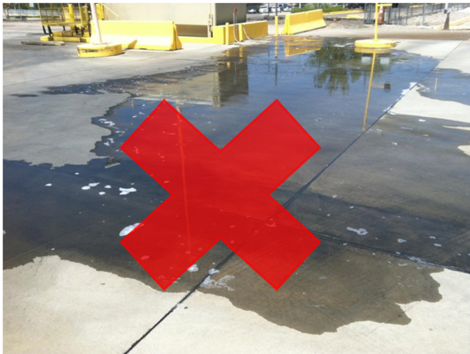
Exhibit A: Higher Risk for Stormwater Impact: Unattended spill
