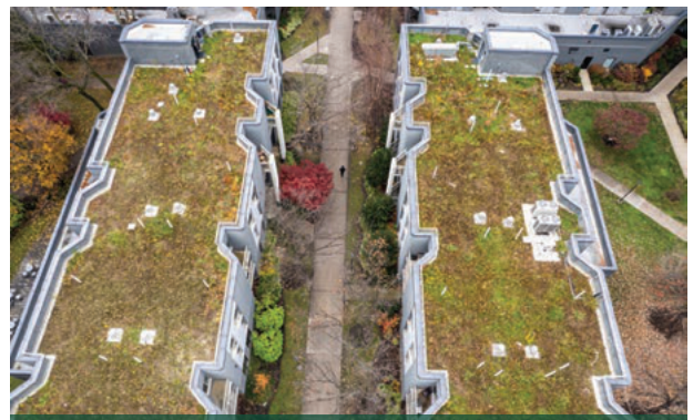
Green Roof - Constructed
