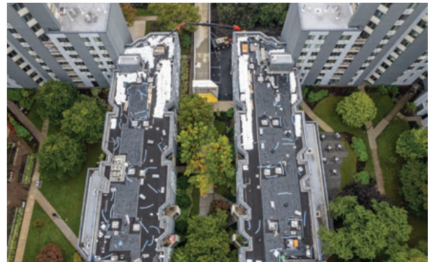
Green Roof - In Construction
