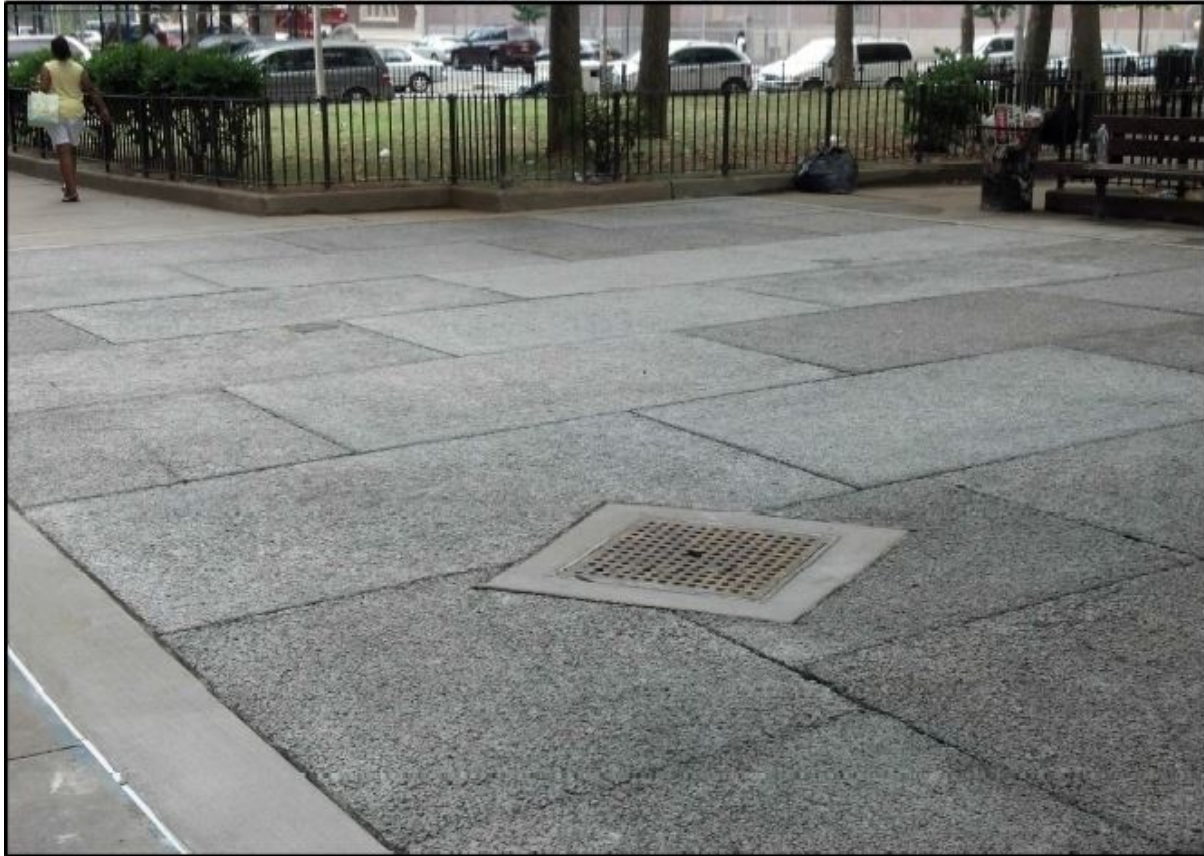
Figure 3-14: Demo Area 2 Porous Concrete Panels and Inlet Grate at NYCHA’s Seth Low Houses
