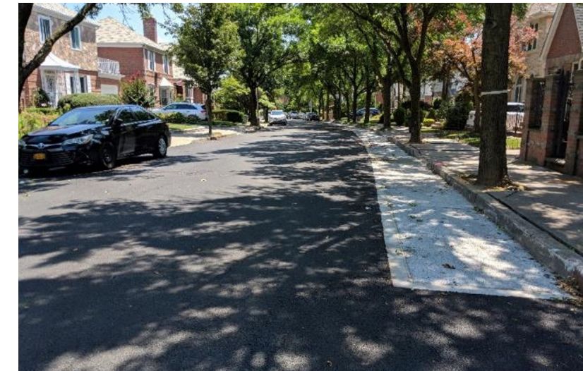
A FINISHED POROUS PAVEMENT INSTALLATION IN QUEENS.
