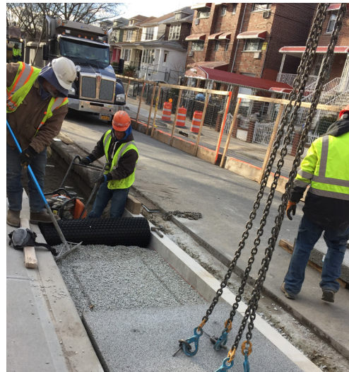
CONTRACTORS INSTALL POROUS PAVEMENT IN THE ROADWAY
