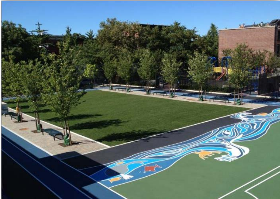
Figure ES-2. PS 261, Brooklyn, School Yard Retrofit (Turf Field/Subsurface Retention, Rain Garden, Porous Pavement)
