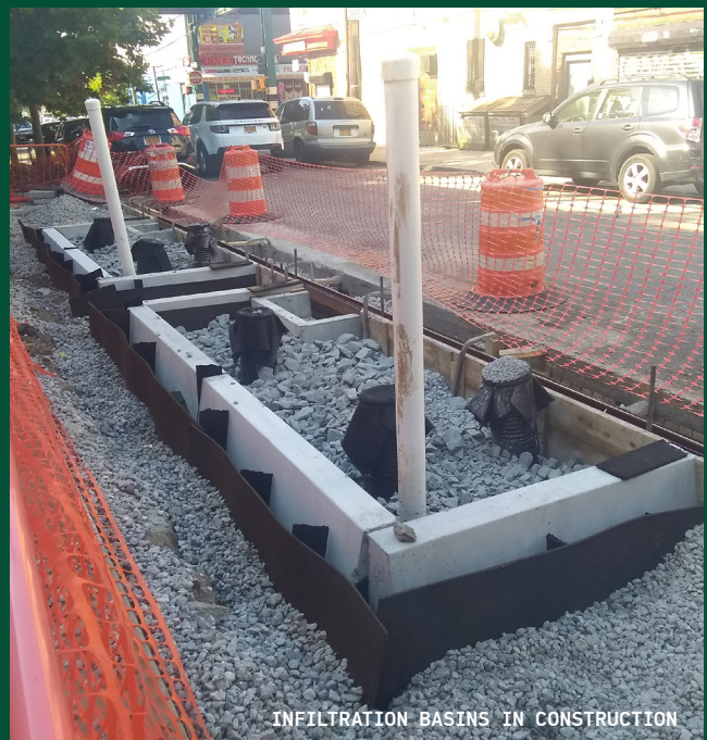
EXCAVATED SITE WITH GEOTEXTILE FABRIC
