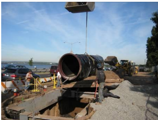
New Sewer Construction
