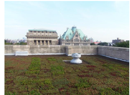
Green Roof Installation
