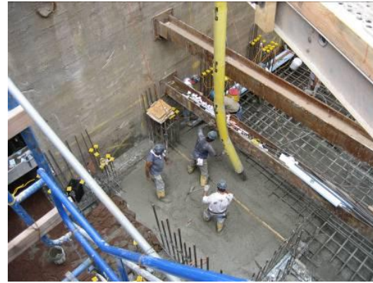
Pump Station Expansion
