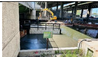
Inspection photo from 8/25/2025 showing construction activity.
