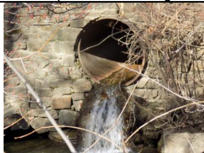
Dry weather discharge observed from the unidentified northernmost outfall in Westchester near S61 Sentinel station in March 2025
