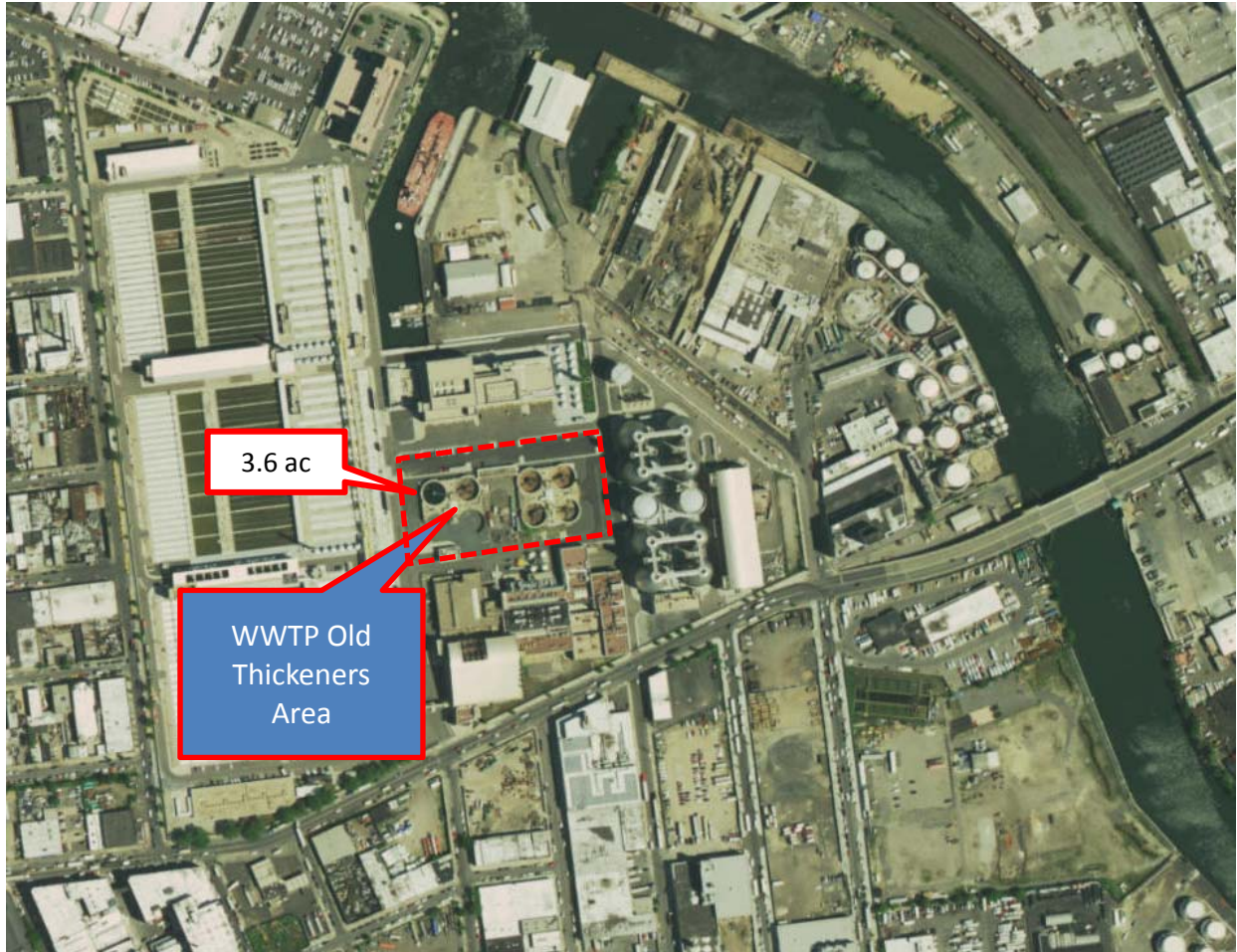
Figure 8-14. Potential Mining Shaft Site near the Newtown Creek WWTP
