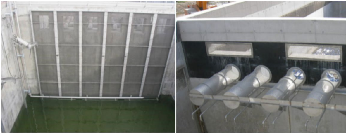
Figure 14 - Retention screens installed in activated sludge aeration basins (Veolia)
