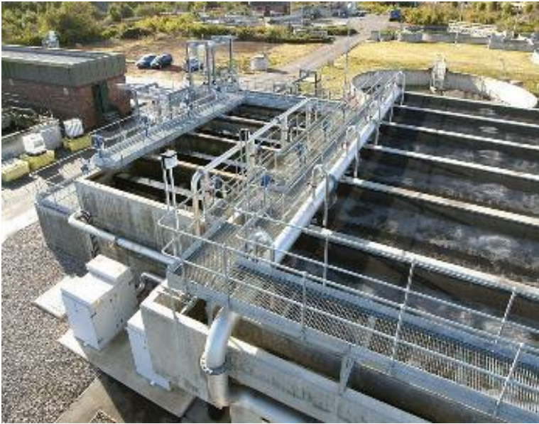
Figure 7 - Example of BAF installation (De Nora's website)
