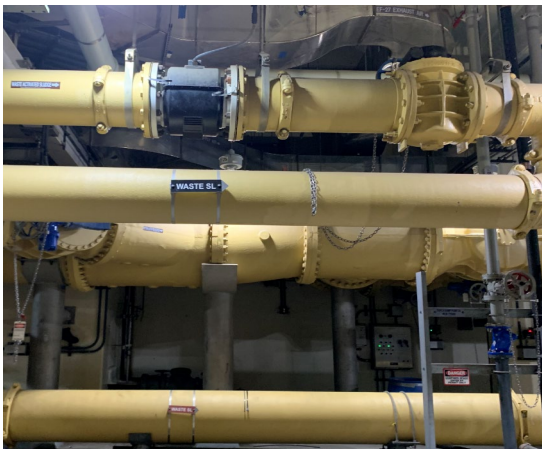
Photo 22 - RAS and WAS Piping are in good condition.
