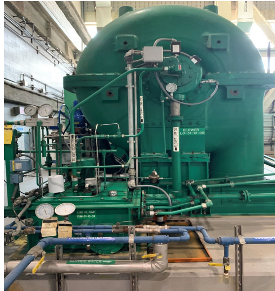
Photo 63 - Process Air Blowers and supporting systems (i.e., lube oil, cooling water, etc) are considered in good condition.
