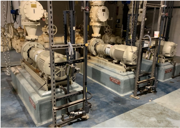
Photo 7 - Scum Recirculation Pumps are in good condition and operating as intended.
