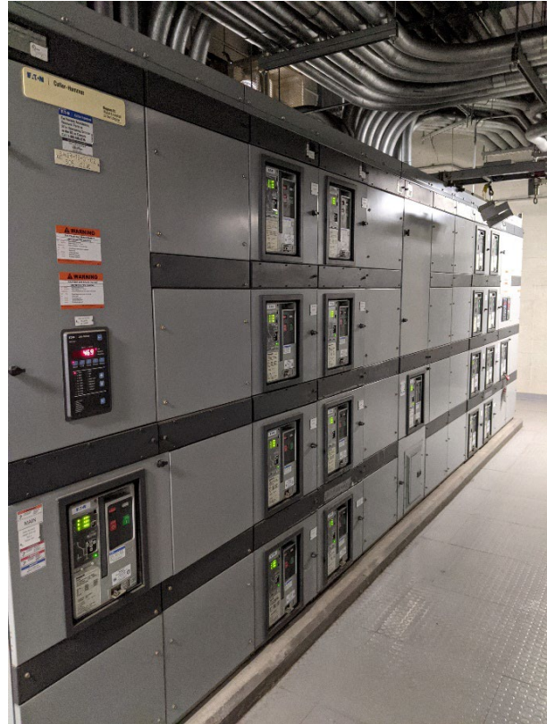
Photo 45 – Switchgear 19-01-02 is in good condition operating as intended.
