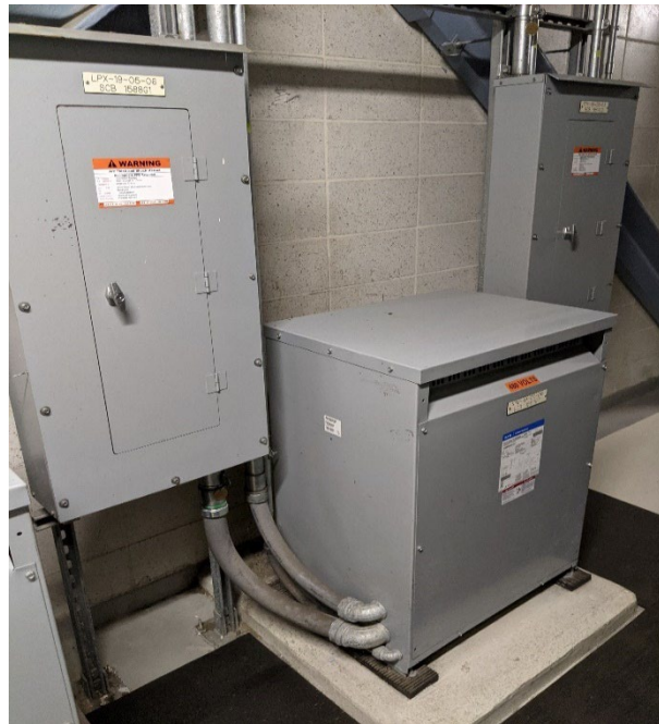
Photo 53 – Transformer is in good condition and operating as intended.
