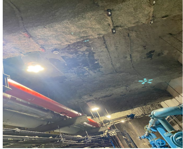
Photo 19 - Ceiling Plaster has detached.
