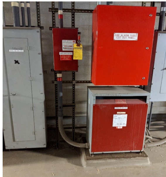
Photo 41 – Fire Alarm Transformer is in good condition with no holes or dielectric leak.
