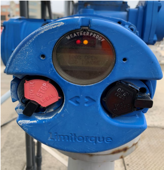
Photo 62 – Rotork actuators were reported to have had significant issues with waterproofing. Actuators will be recommended for replacement for each BNR alternative assesses.
