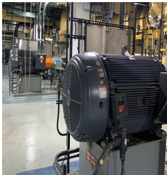
Photo 25 - RAS Motors are in good condition.
