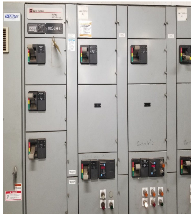
Photo 57 – MCCs devices are functional and MCC is in good condition.
