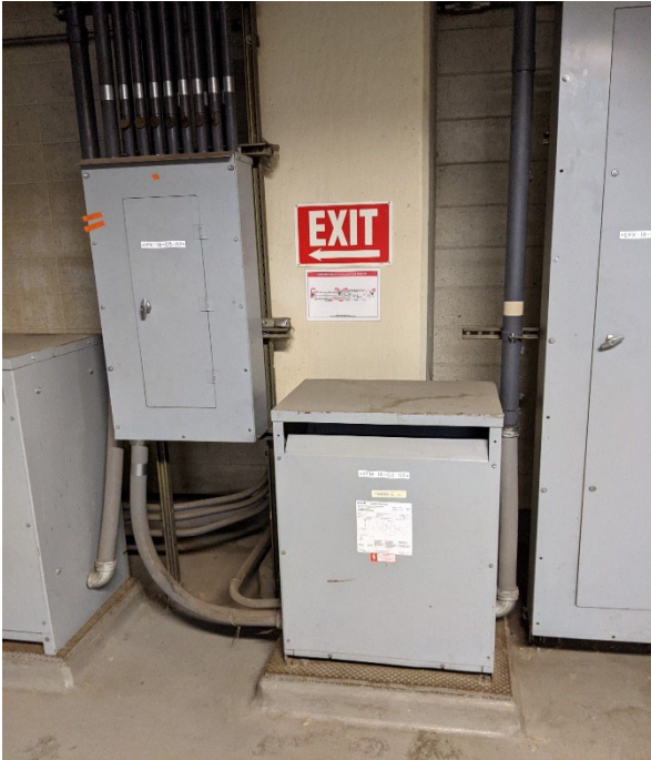
Photo 38 – Transformer is in good condition with no holes or dielectric leak.
