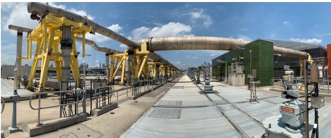
Photo 11 - Process air header over to South, Central and North Batteries appears in good condition. Structural was able to assess the support structure throughout the batteries and confirmed its in good condition.
