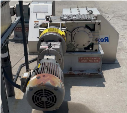
Photo 26 - Surface Corrosion on motor noted but unit is still in good condition, operating as intended.
