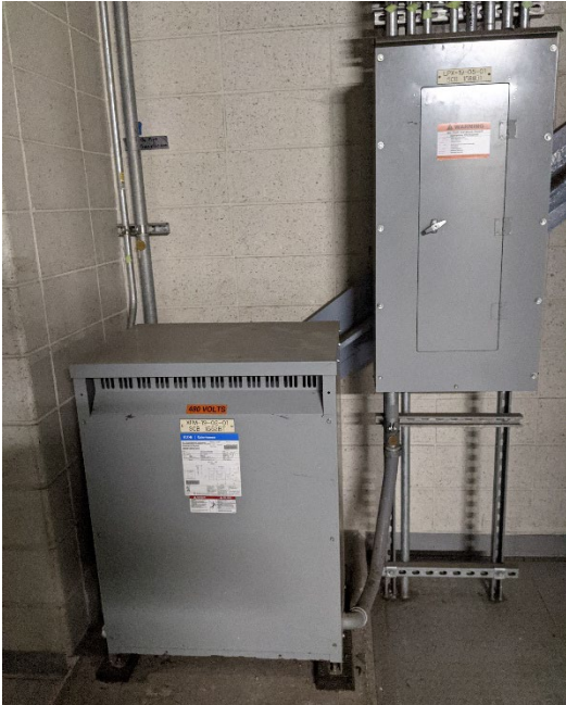
Photo 50 – Transformer is in good condition and operating as intended.
