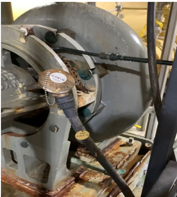
Photo 24 - RAS Pumps are mostly in good condition. RAS pumps #3 had significant leakage during our assessment. Corrosion, likely caused by the leak, was noticed as well.
