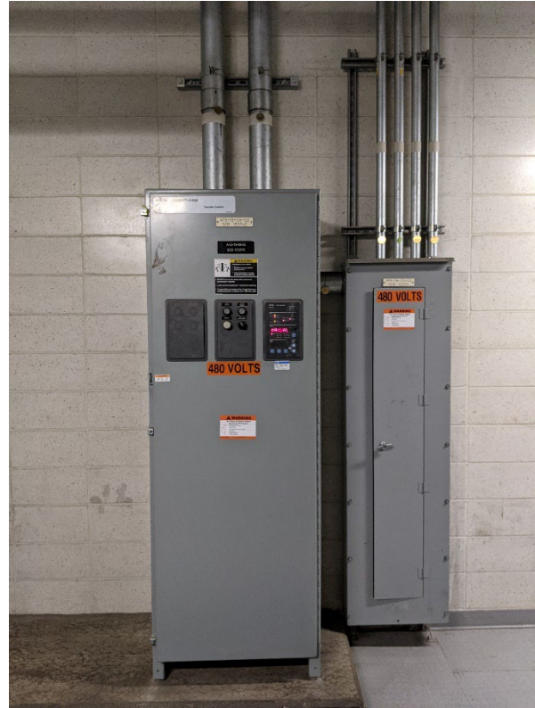
Photo 49 – ATS is in good condition and operating as intended.
