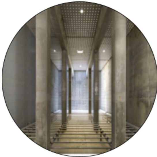
Interior of BIOSTYR Cell
