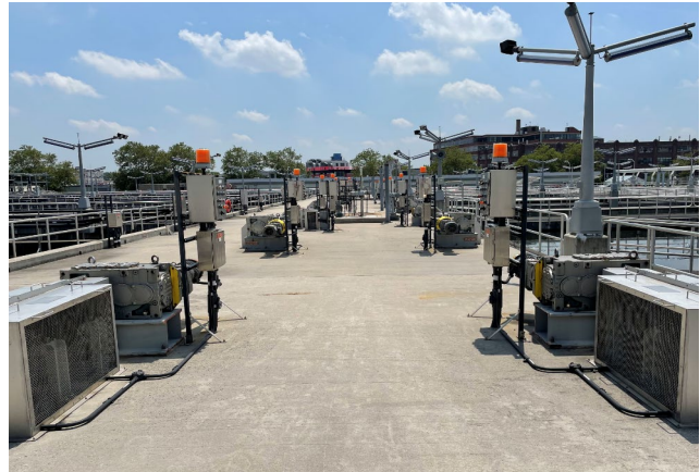
Photo 27 - All cross and Longitudinal collector drives are considered in fair to good condition.
