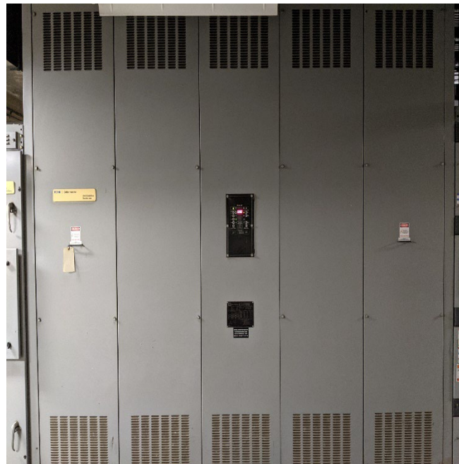
Photo 32 – Unit Substation Transformer have cover doors and limited view of the inside connections.
