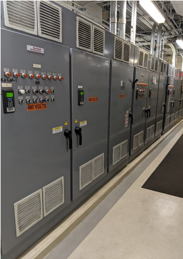
Photo 54 – VFD #1, VFD #2, VFD #3, and VFD #4 are in good condition operating as intended.
