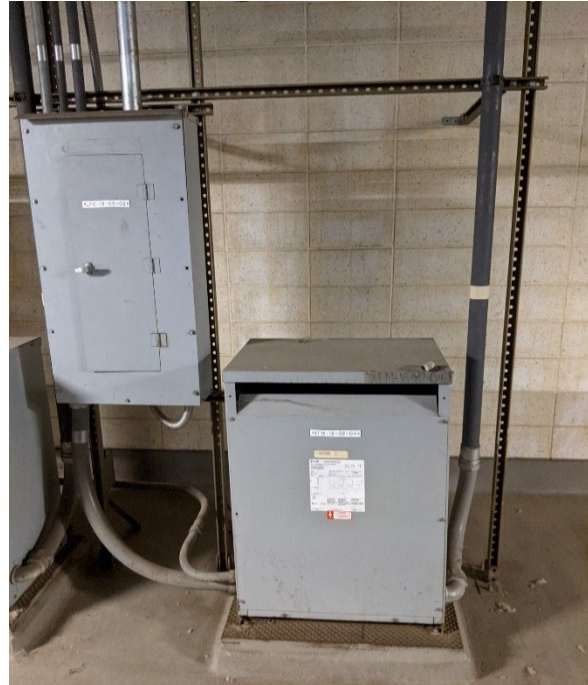
Photo 39 – Transformer is in good condition with no holes or dielectric leak.
