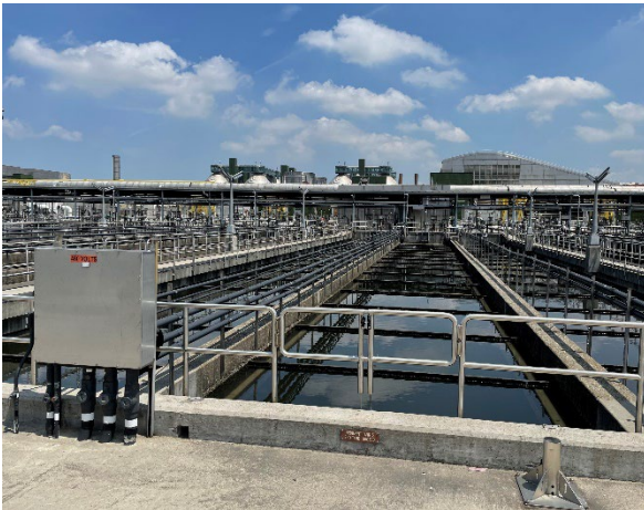
Photo 28 - Skimmings collection atop each tank was operating as intended.
