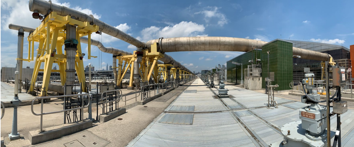
Photo 66 - Process air header over to South, Central and North Batteries are in good condition. Both process mechanical and structural team members assessed the system and confirmed it is in good condition.
