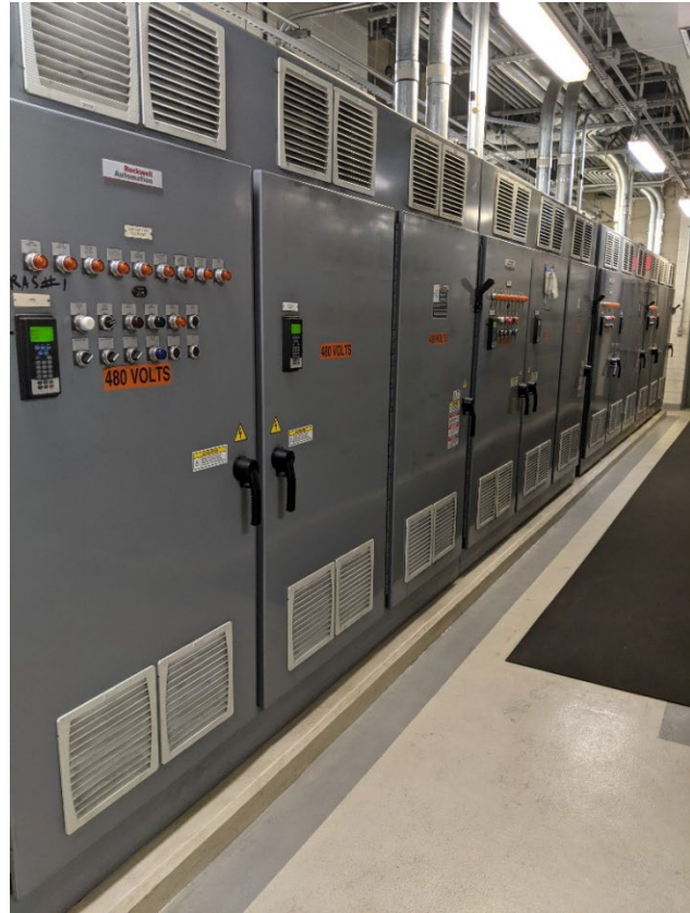
Photo 61 – VFD #1, VFD #2, VFD #3, and VFD #4 appear in good condition operating as intended.
