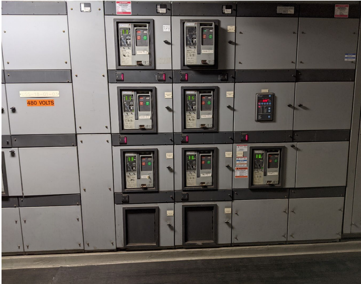
Photo 33 – Unit Substation overall rating is in good condition.
