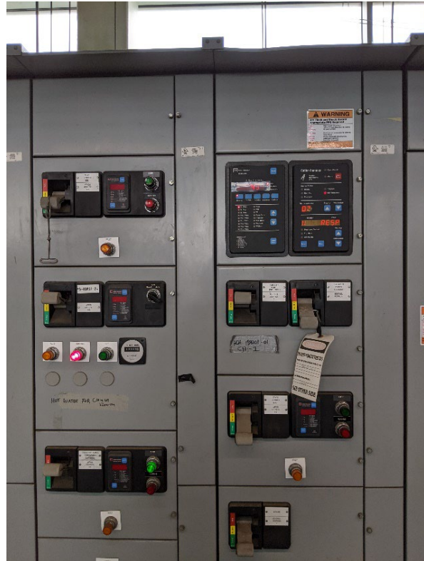
Photo 35 – Devices are functional, one MCC cubicle lockout of service.
