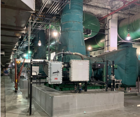
Photo 18 - Odor Control Fans in good condition. Carbon Tanks at surface level operating as intended.
