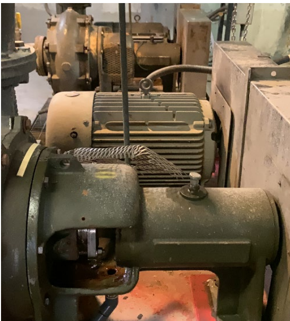
Photo 3 - Several of the grit pumps in the North Battery were leaking during our inspection.
