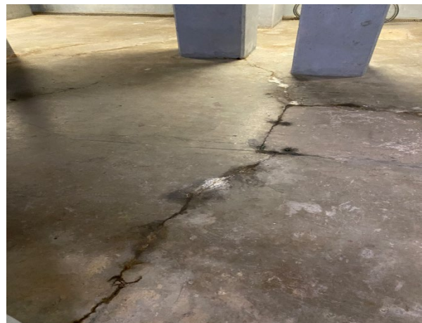
Photo 17 - Lower level/Tunnel level floor cracks that have been fixed.
