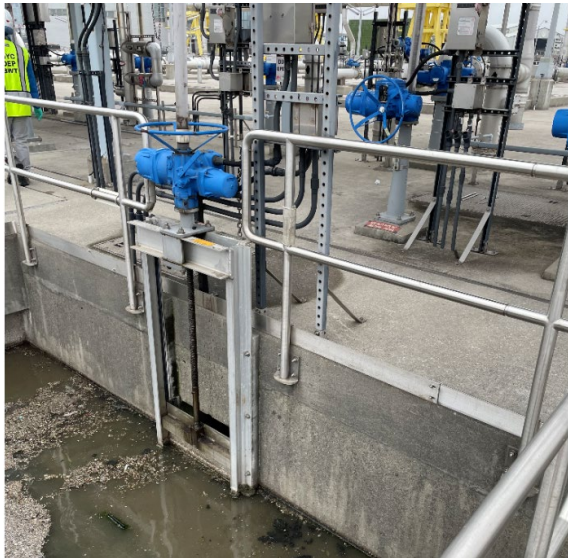
Photo 5 - Scum Collection System in good condition and operating as intended.
