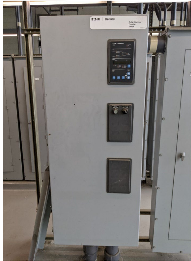
Photo 37 – ATS switch is in good condition, no label or tag to identify the system.
