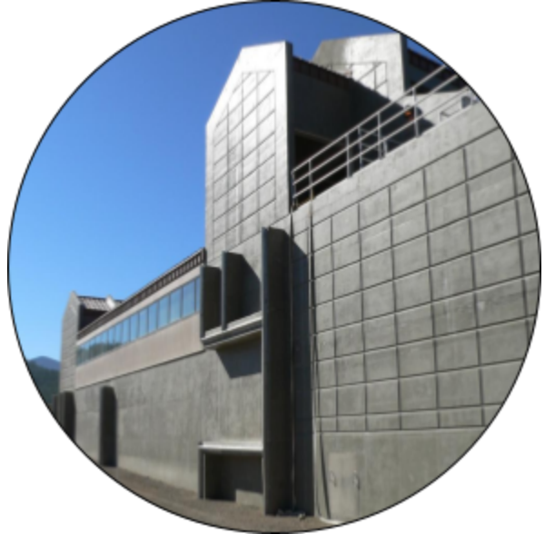
10 MGD Tahoe-Truckee SD BIOSTYR - Truckee, CA
