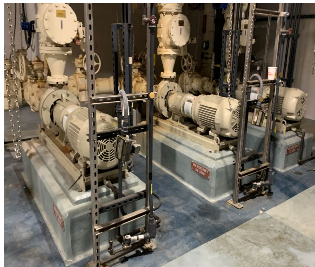
Photo 65 - Skimming Transfer and Recirculation chopper pumps are in good condition.
