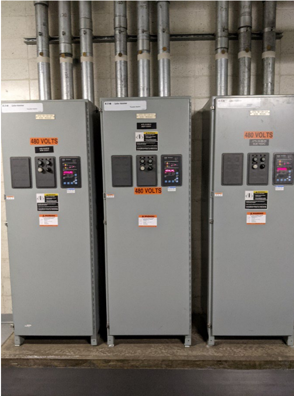
Photo 48 – ATS is in good condition and operating as intended.
