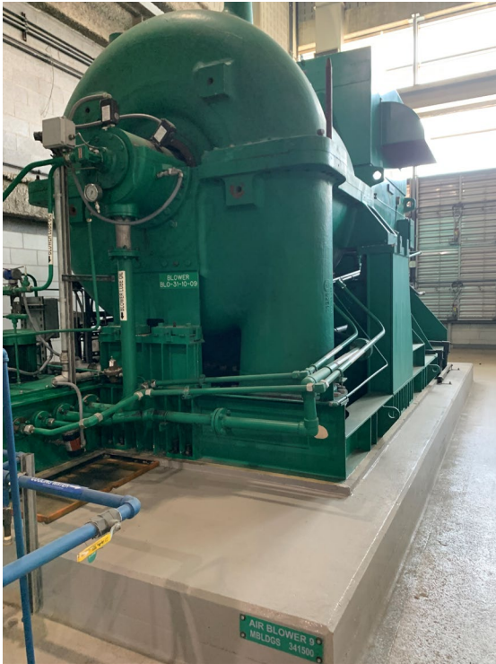
Photo 9 - Process Air Blower in good condition, operating as intended.
