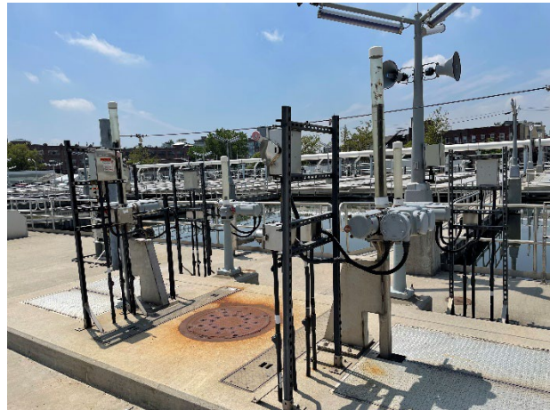
Photo 29 - Rotork actuators are older compared to Central and North Batteries. As noted by DEP, there have been issues with Rotork actuators in the past. These are considered in fair condition, but water infiltration could cause operational issues.
