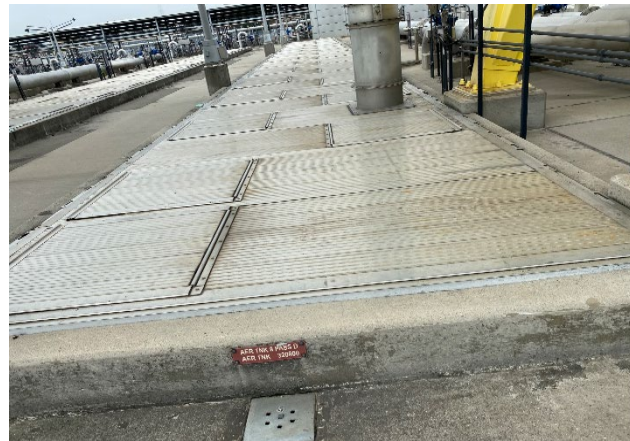
Photo 15 - Condition across all three batteries is consistent. Tanks are considered in good condition.
