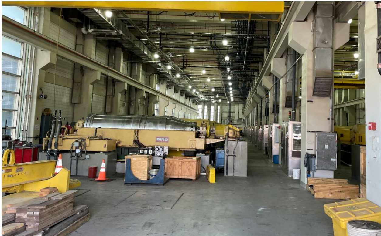
Photo 30 – Centrifuges located in the Thickener Building, are in good condition.
