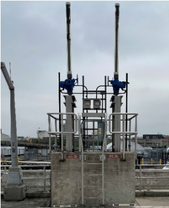
Photo 1 - Grit uptake shaft, with two sluice gates, permits flow into one of two grit tanks. Shafts are in good condition.
