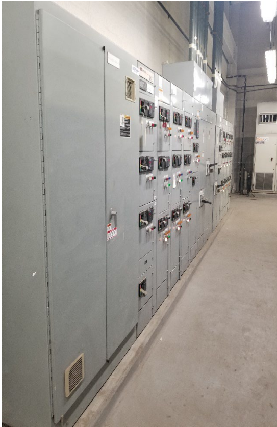
Photo 60 – Motor Control Centers in both the North and South Control Building Electrical Rooms are in good condition.
