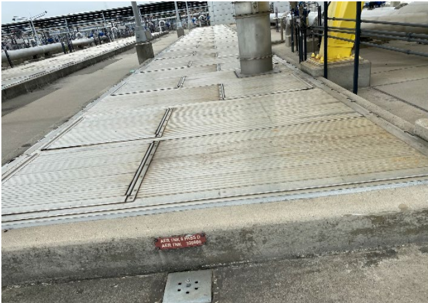
Photo 58- Aeration Tanks, shown above, were covered in aluminium cladding. The visible portion of the tanks and cladding are considered in good condition.
