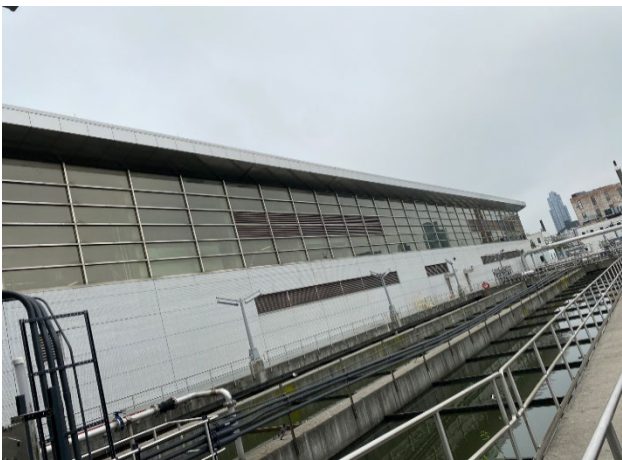
Photo 16 - Control Buildings are considered in good condition.
