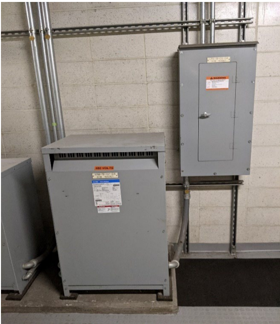
Photo 52 – Transformer is in good condition and operating as intended.
