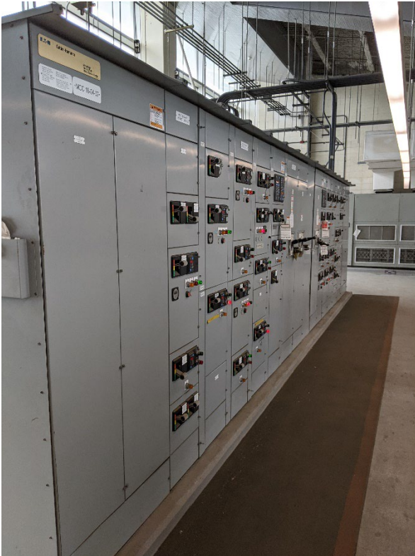
Photo 34 – MCC 18-04-03 unit appears in good condition operating as intended.
