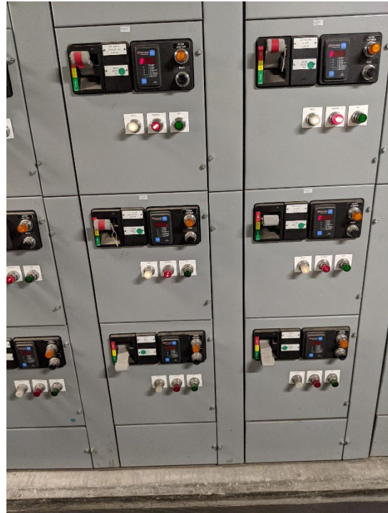
Photo 47 – MCCs is in good condition.
