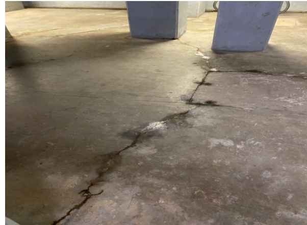
Photo 59- Settling Cracks in the tunnel system were noted during our assessment. The facility has already taken the proper measures to secure these cracks.
