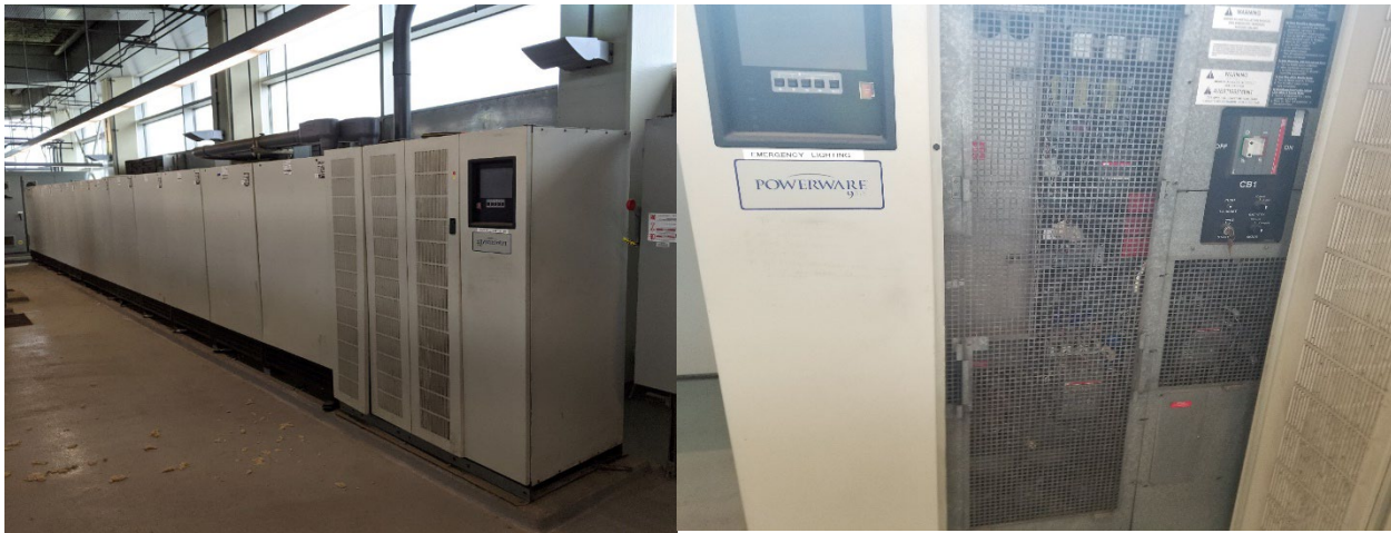
Figure 3-13: Newtown Creek WRRF – Site Photographs of UPS in Electrical Room in North Battery Building
