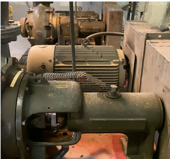
Photo 64 - Several grit pumps in the North Battery were visibly leaking during our inspection. The condition of the pump support pads was noticeably corroded, likely due to pump leakage. These pumps are considered in fair condition currently, but likely will deteriorate quickly.
