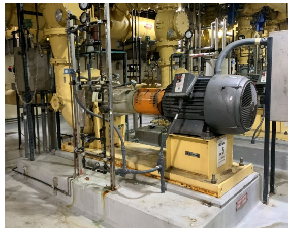
Photo 23 - WAS Pumps are in good condition. Some corrosion was noticed on the system; however, it does not impact operations.
