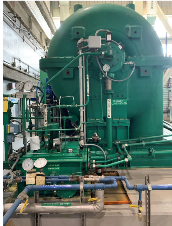
Photo 10 - Process Air support systems, cooling water and lube oil, both appear to be in good condition without operating issues.
