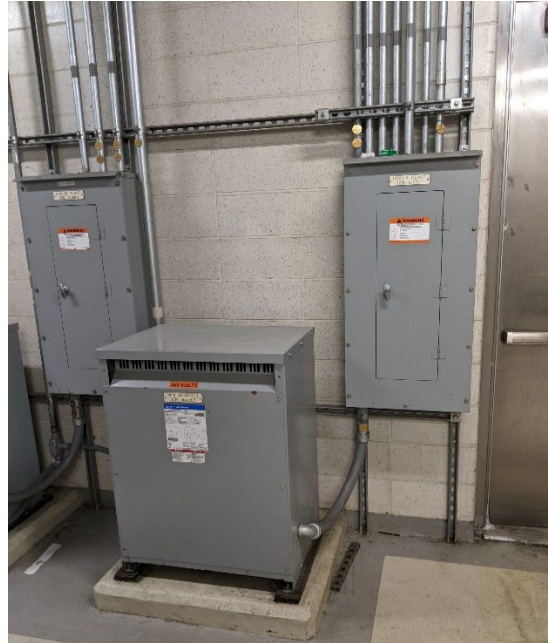
Photo 51 – Transformer is in good condition and operating as intended.
