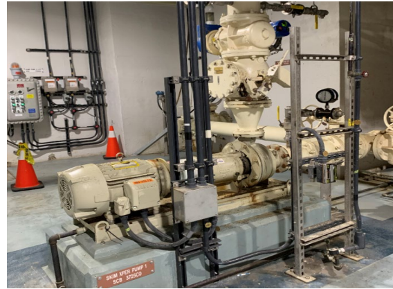
Photo 8 - Scum Transfer Pumps are in good condition and operating as intended.
