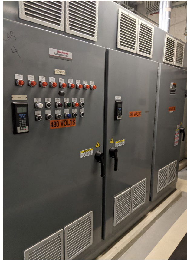
Photo 55 – VFD #4 is in good condition operating as intended.
