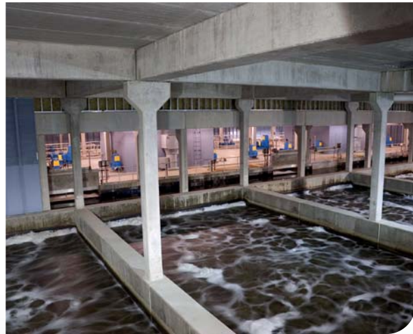
Treated effluent at top of cells
