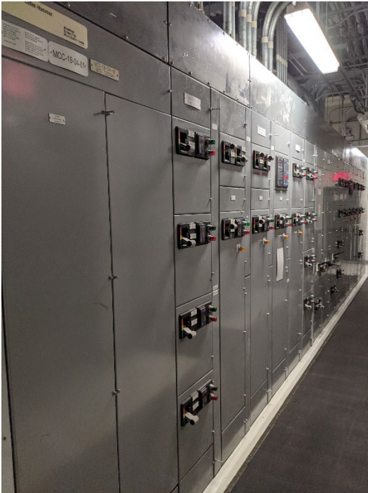
Photo 46 – MCC 19-04-01 unit is in good condition operating as intended.
