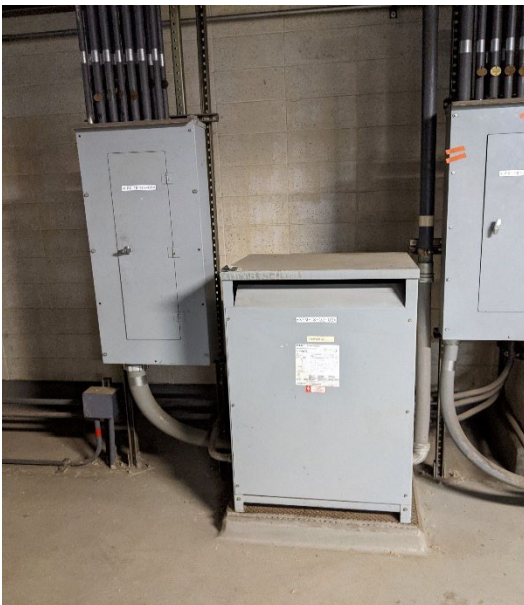
Photo 40 – Transformer is in good condition with no holes or dielectric leak.
