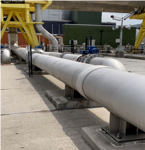
Photo 12 - Process Air piping into each tank seemed in good condition, with no reported issues or clear leaks.
