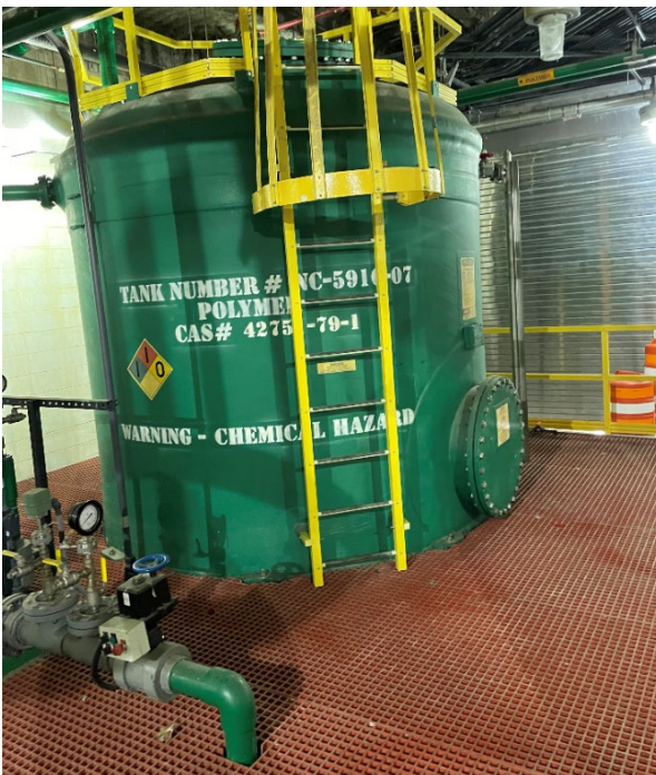
Photo 20 - Polymer Storage Tanks are in good condition
