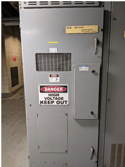
Photo 31 – Unit Substation Disconnect Mechanism have cover doors and limited view of the inside connections.
