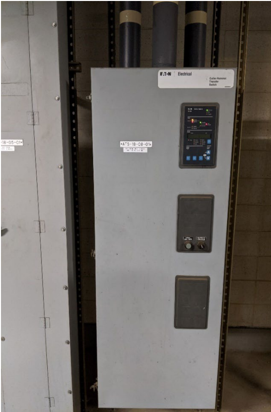
Photo 36 – ATS is in good condition, and is operating as intended
