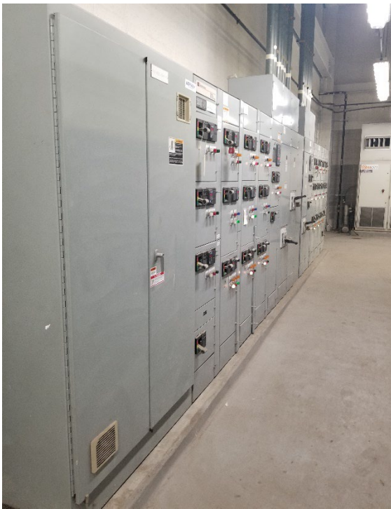
Photo 56 – MCC is in good condition operating as intended.
