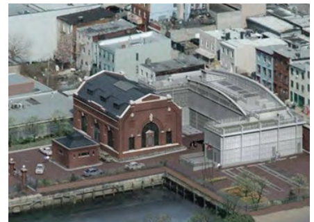
Gowanus Pumping Station
