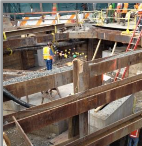
Trenching to Install New Whitestone Interceptor Near TI WWTP
