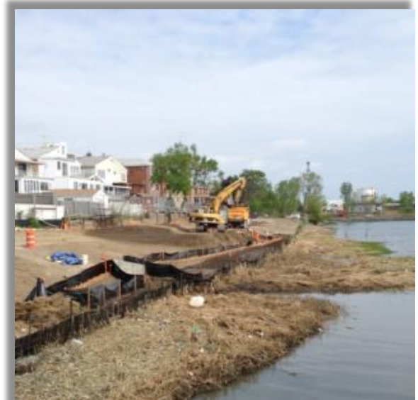
New Interceptor Route Being Restored to Upland / Wetland
