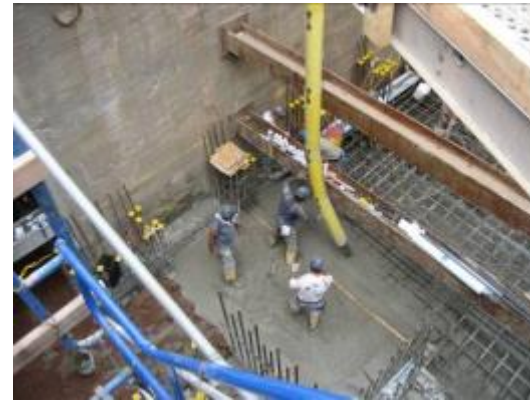
Pump Station Expansion
