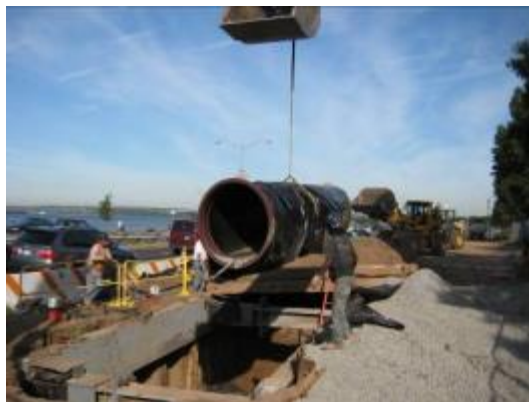
New Sewer Construction
