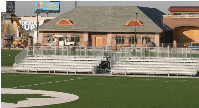
CSO Storage Facility
