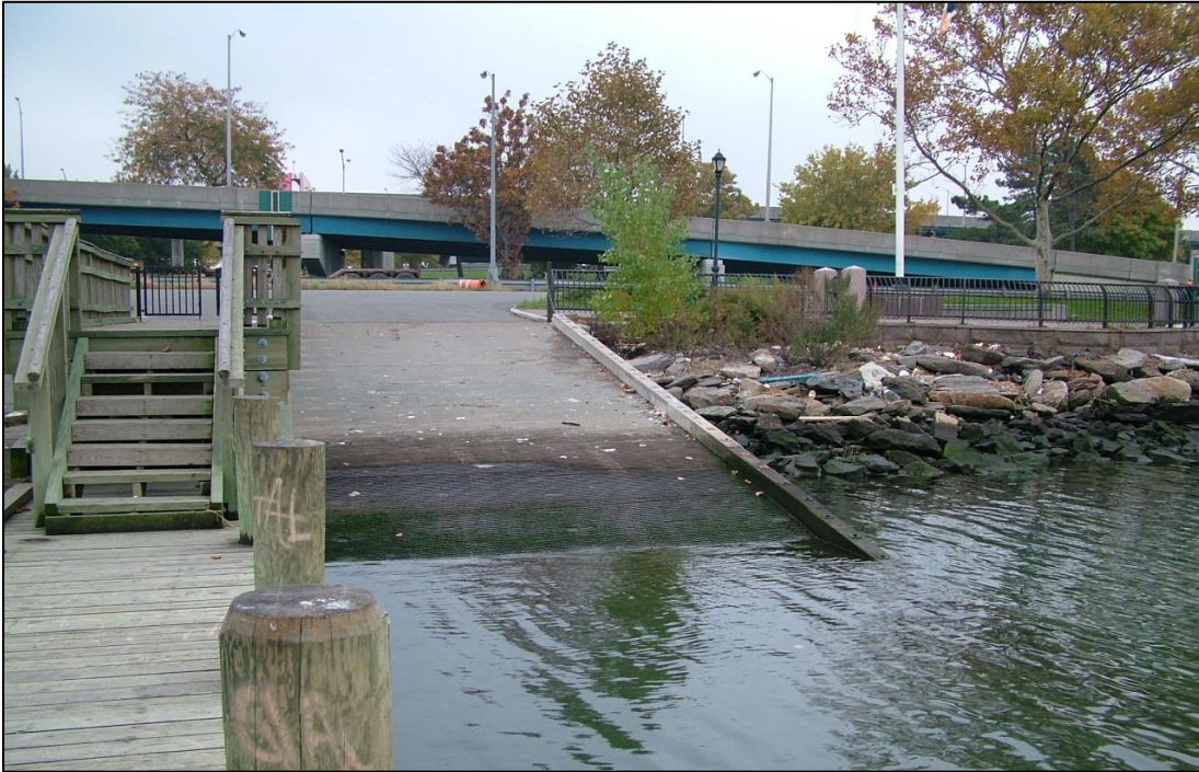
Figure 2-23. Boat/Kayak Launch at the East End of Flushing Bay Promenade
