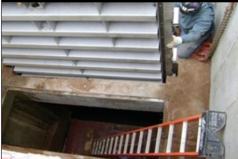
1 Port Richmond WWTP Throttling Facility
