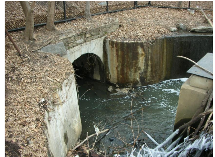
Entrance to collection system
