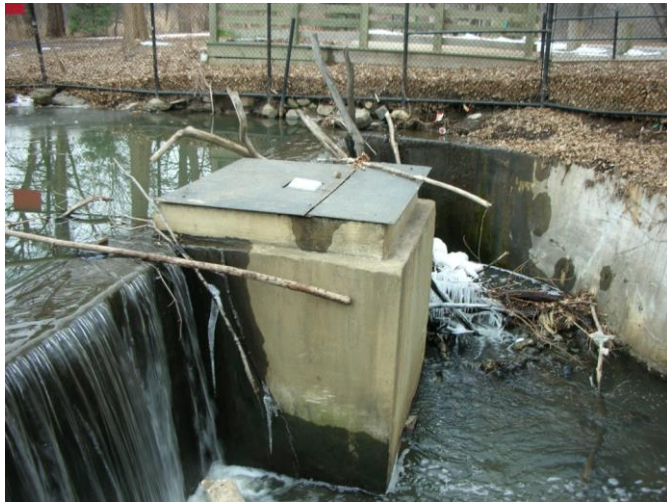
Overflow weir structure
