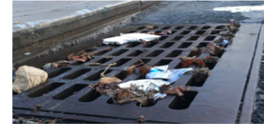
■ Catch Basin Hooding
