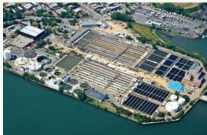
Wastewater Resource Recovery Facility (WRRF)
