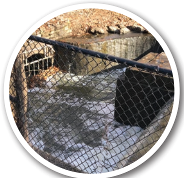
Existing outlet structure
