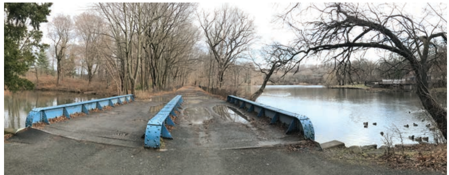
Southern end of Van Cortlandt Lake near outlet structure
