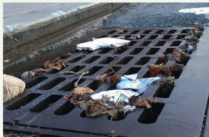
Catch Basin Hooding
