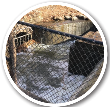
Existing outlet structure
