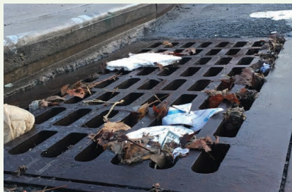
Catch Basin Hooding
