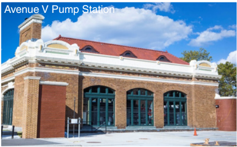
Avenue V Pump Station
