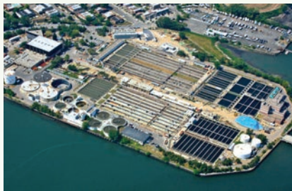
Wastewater Resource Recovery Facility (WRRF)
