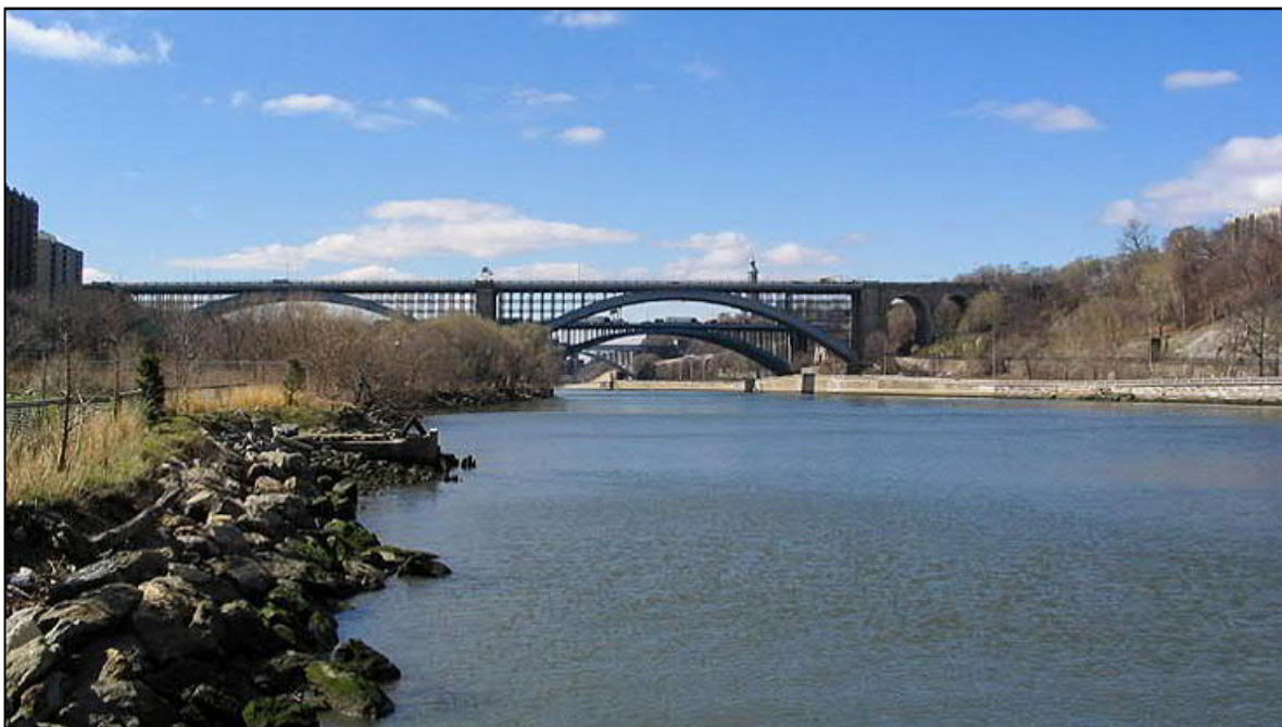
Figure 2.1-22. Riprap and Bulkhead Shoreline of Harlem River
