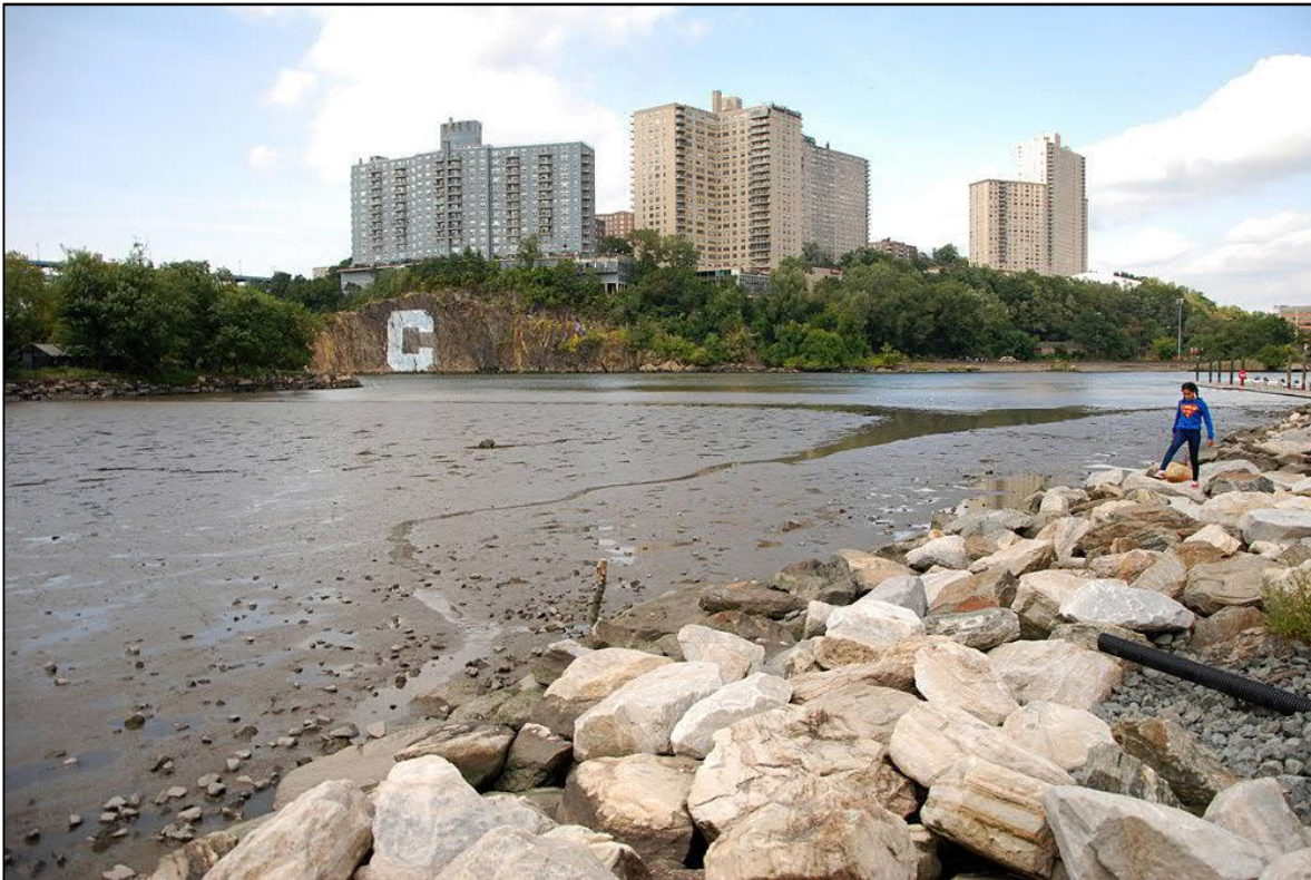
Figure 2.1-21. Riprap and Natural Shoreline View of Harlem River
