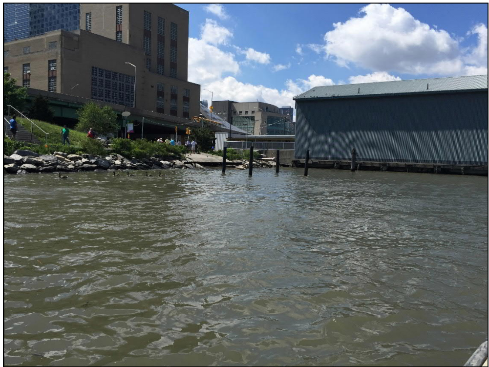
Figure 2.2-21. Rip Rap and Pier Shoreline of Hudson River
